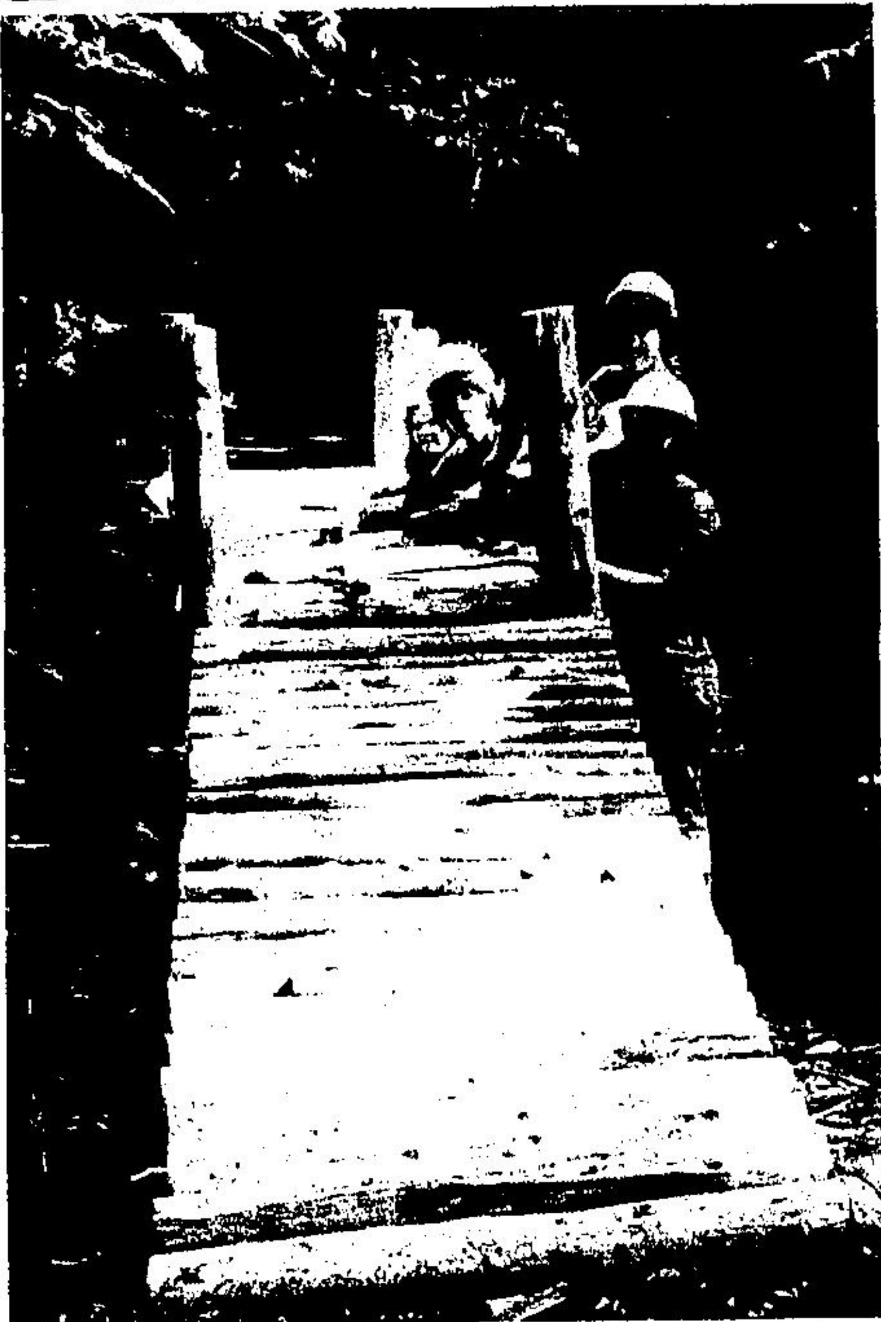
CONSTRUCTING a foot bridge across the Black Creek in the Limehouse Conservation Area are Debbie Mason, Hamilton; Caroline Cussen, Mississauga; Bill Christie, Mississauga; and Linda Bruce, Port Credit. They are Experience '78 workers. Missing from the crew when the picture was taken were Wayne Wolfstadt, Toronto; Mark Partridge, Mississauga; Chris Halliday, Mississauga.
