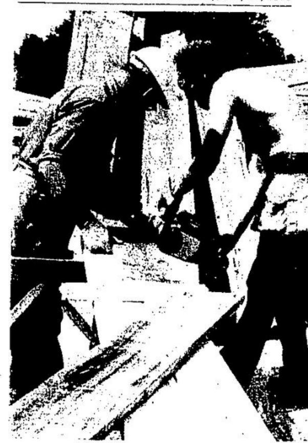
THE NEW with the old. Doug Robertson, builder of log houses and barns, uses a chain saw with Stan Robinson's help. The Eden Mills resident fisishes construction with authentic broad axes, adzes and chisels. The crew are working on reerecting a log barn in Nassagaweya.
