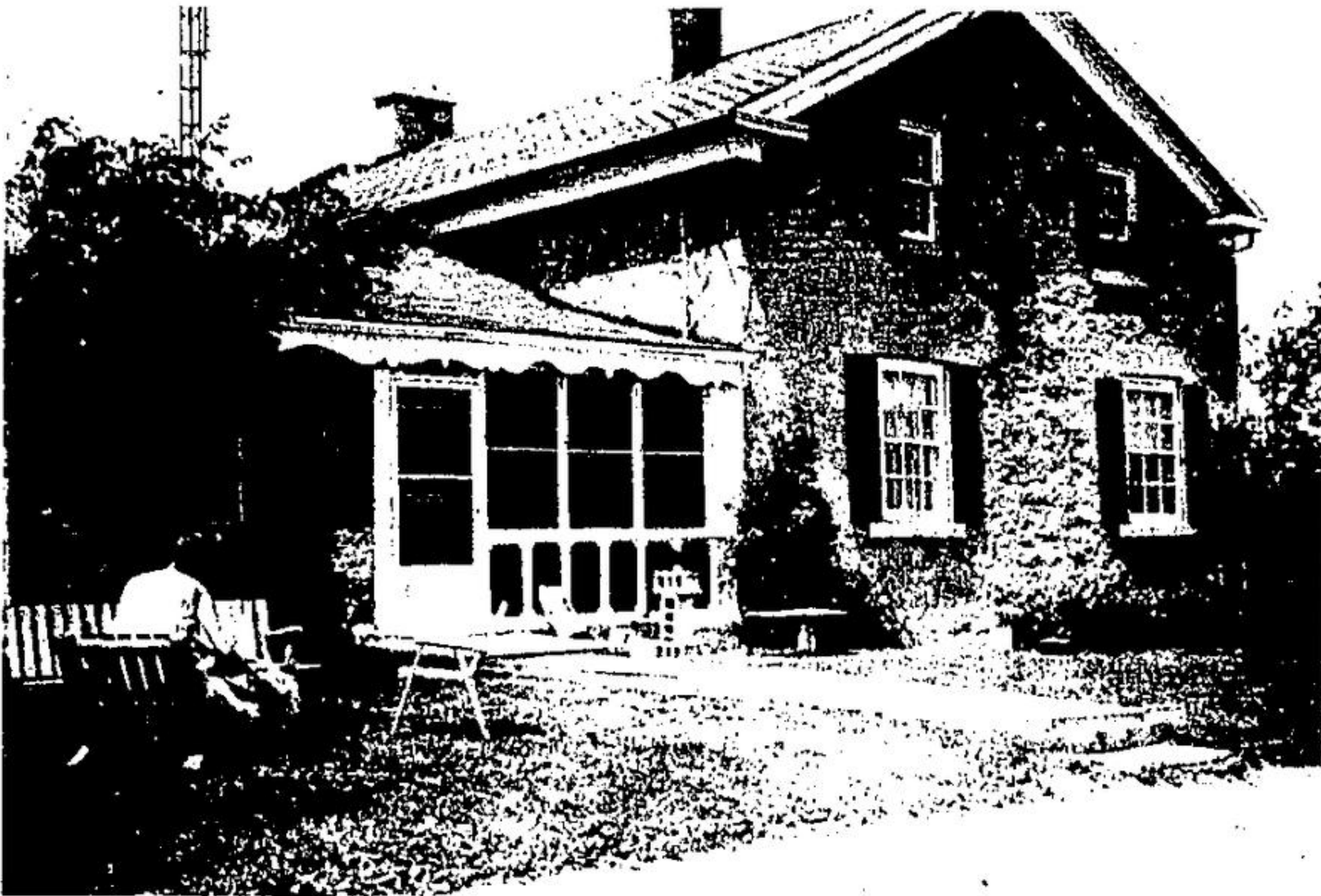
RENOVATING A STONE farm house means lots of hard work, but Mike and Joan Silk are having fun refurbishing their Ospringe home. Shutters
