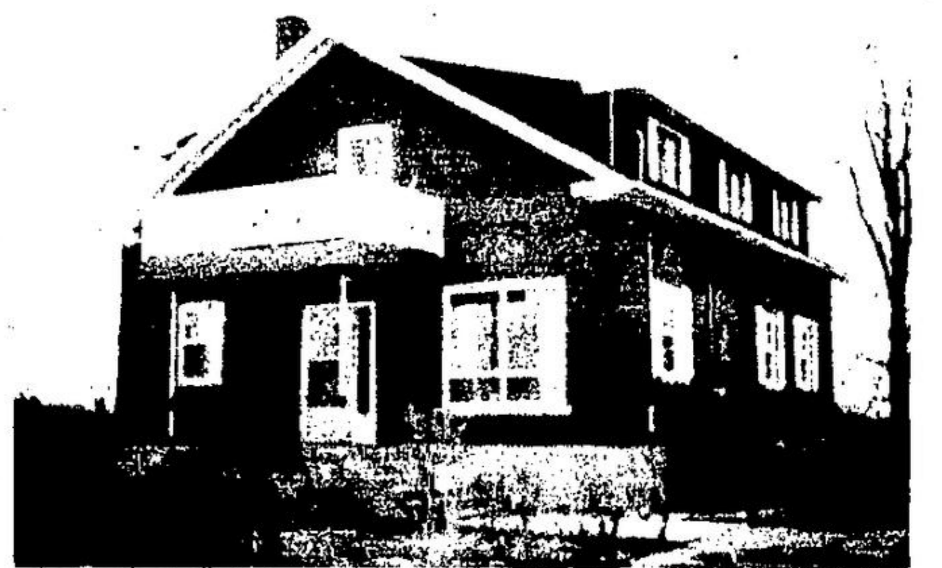
NOW A MODERN home, old Dublin school has gone through many changes in past years. In the conversion, a side window was bricked up, the belfry removed and a second story added. It is now the home of Mr. and Mrs. Douglas McRae.
