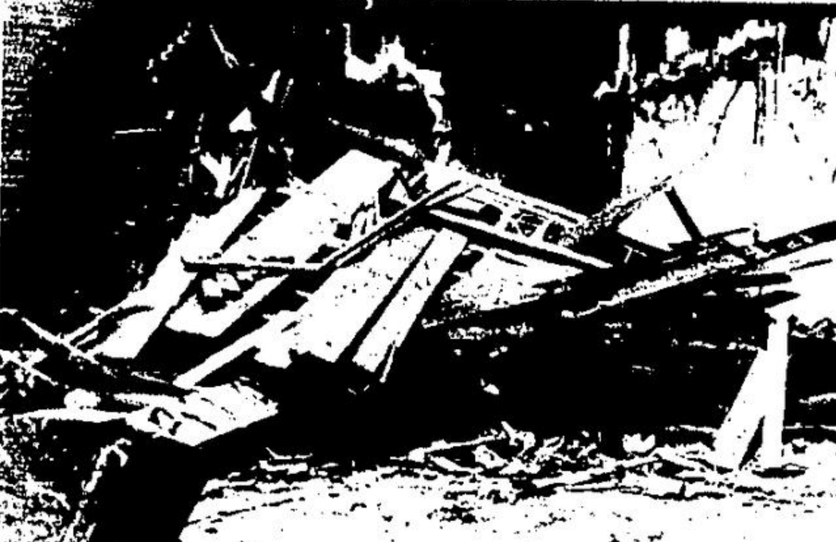
FRAME ADDITION at the rear of Elissa shoe store was razed Tuesday. An addition will be built to replace it. When repairs are made, Elissa Shoe Store will re-open. The Cavics lost their business and home by fire in February.
