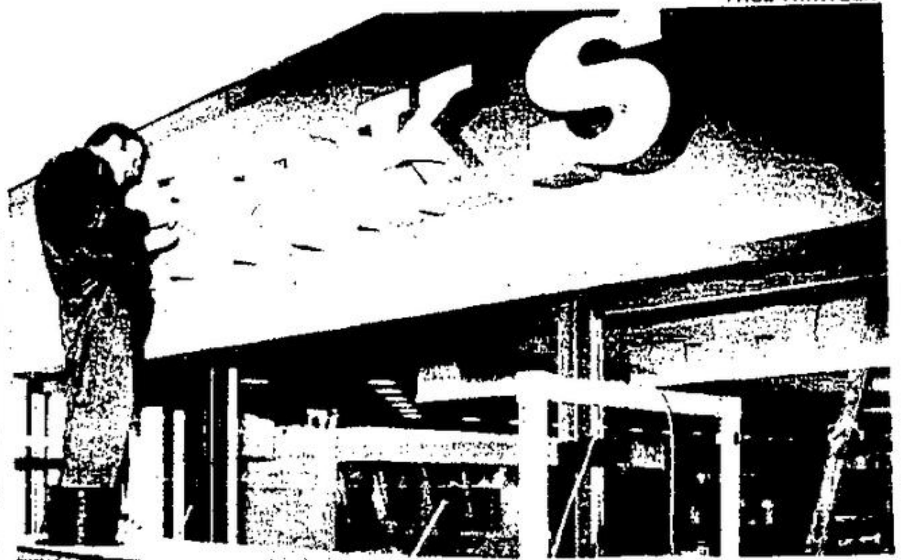
BIRKS SIGN BEING INSTALLED
