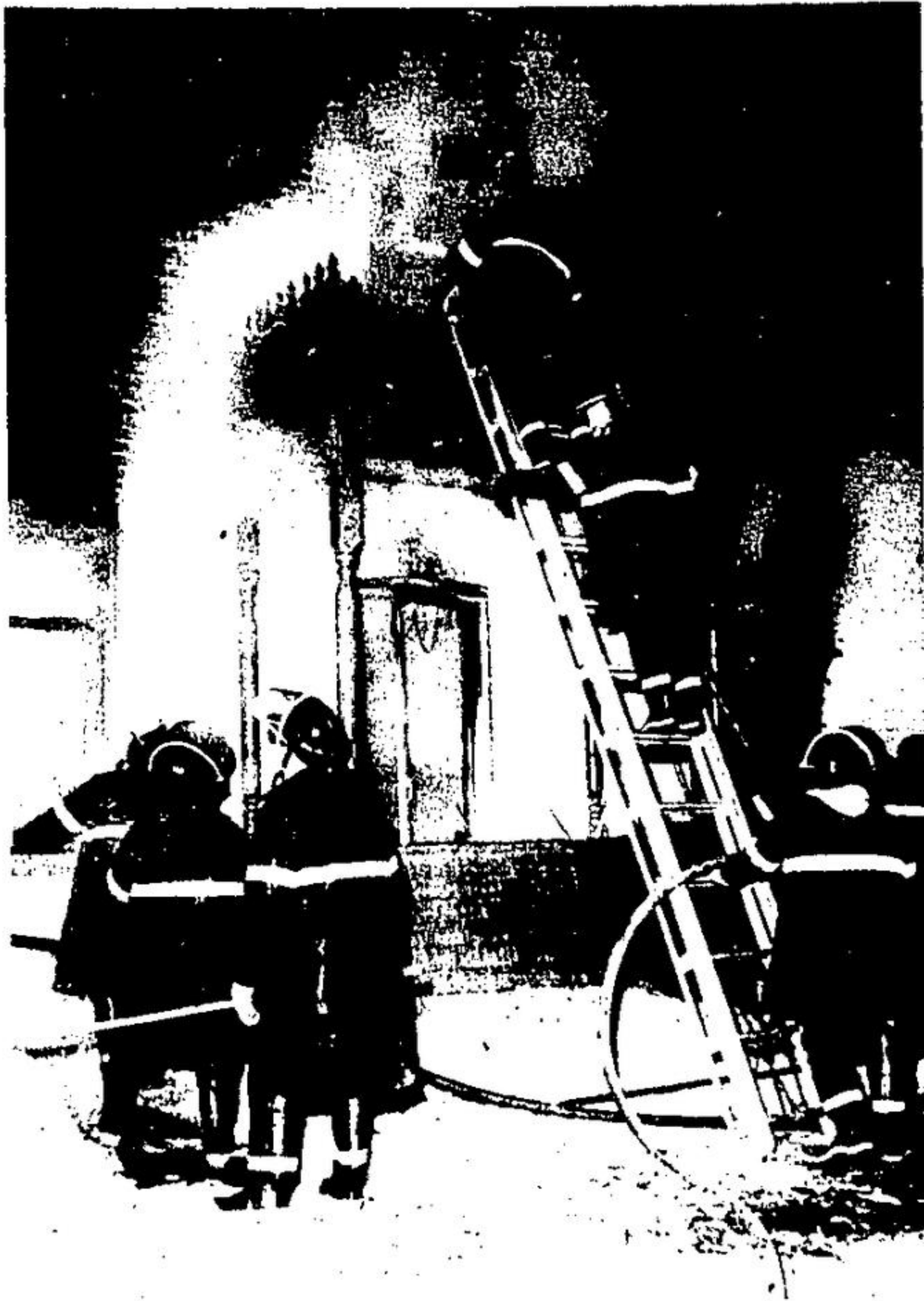
ACTON VOLUNTEER FIREFIGHTERS work frantically to save the Van Merkestein home at 114 Mill St., early last Friday morning. Smoke and flames could be seen all over town in the night sky. In the end, $62,000 damage had been done, and two people were admitted to hospital. The house is beyond repair, according to Fire Prevention officer Larry Brassard.
