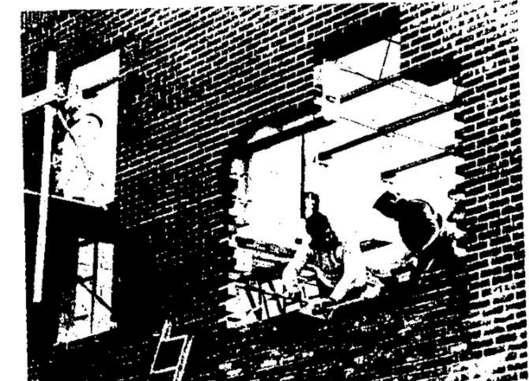
DUE TO AN error , window openings in the fire hall addition must be moved up two feet. Replacing a damaged beam, which was dropped, is delaying other work.
