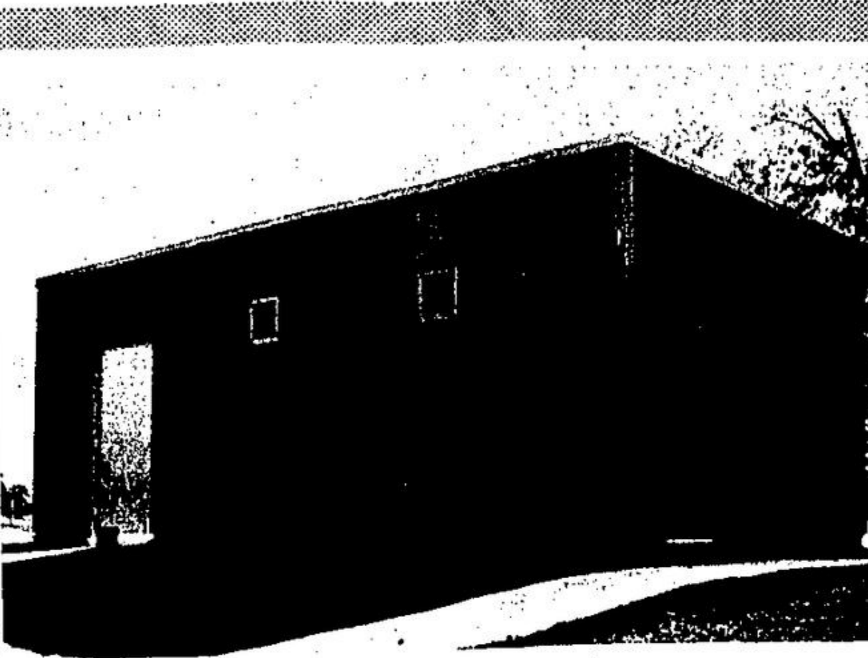
NEW PUMPHOUSE is now in operation at Fairy Lake.
