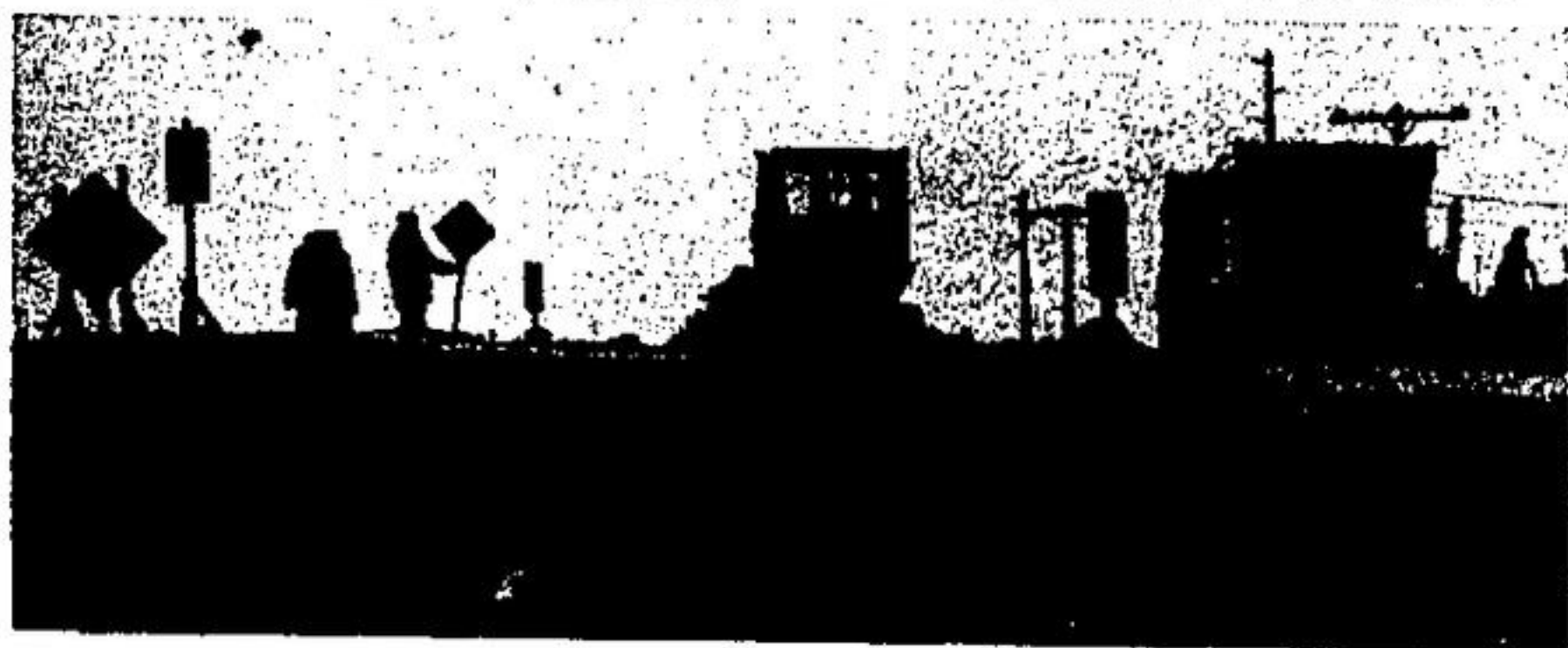
THE SIGN SAYS SLOW and that is what the work has been along highway No. 7. Rain has hampered the construction crews' efforts, dragging the work out beyond its original schedule.
