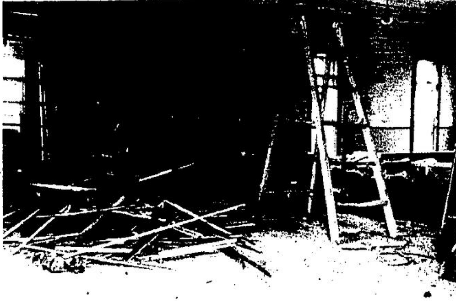
UPSTAIRS AT THE town hall the wreckers have been busy, tearing apart the stage so the addition to the fire hall can be built.
