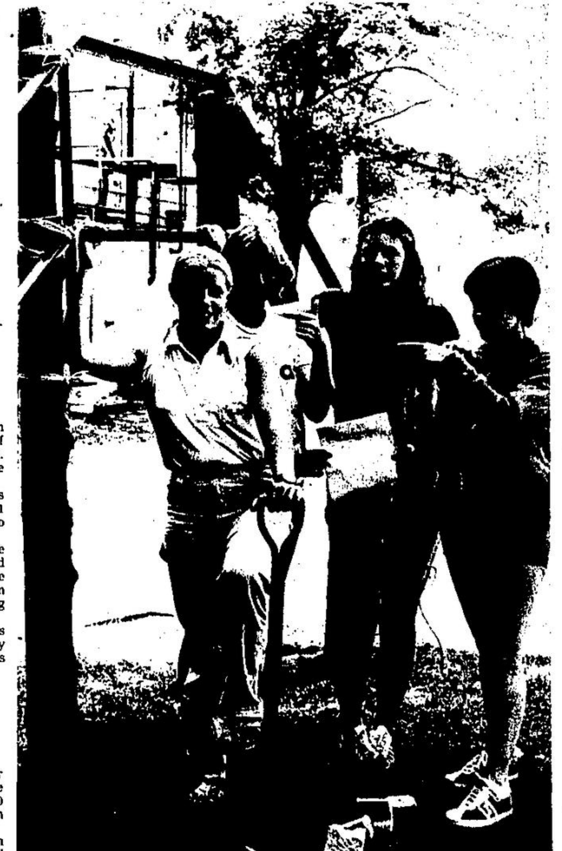
NOW WHAT'S SHE DONE? Sue Mellor, left, seems to be the centre of attention as Ellen Barkman, Karen Glenn and Colleen DeBruyn, (right) point her out. The girls were leaders at the day camp and were building a barn structure for the day camp parents' night Thursday evening.
