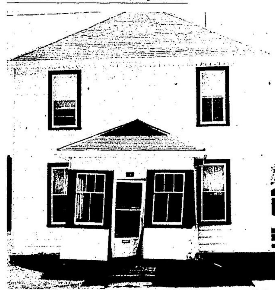
OUT OF SQUARE WITH the rest of Jim Brydon's home on Young St. is his veranda. The veranda has been pushed off its foundations and the windows have been broken and pushed out of square. The aluminum door is bent and the aluminum siding is warped and bent. Police estimate the damage at \$600 but Mr. Brydon's insurance company has yet to make its report.
