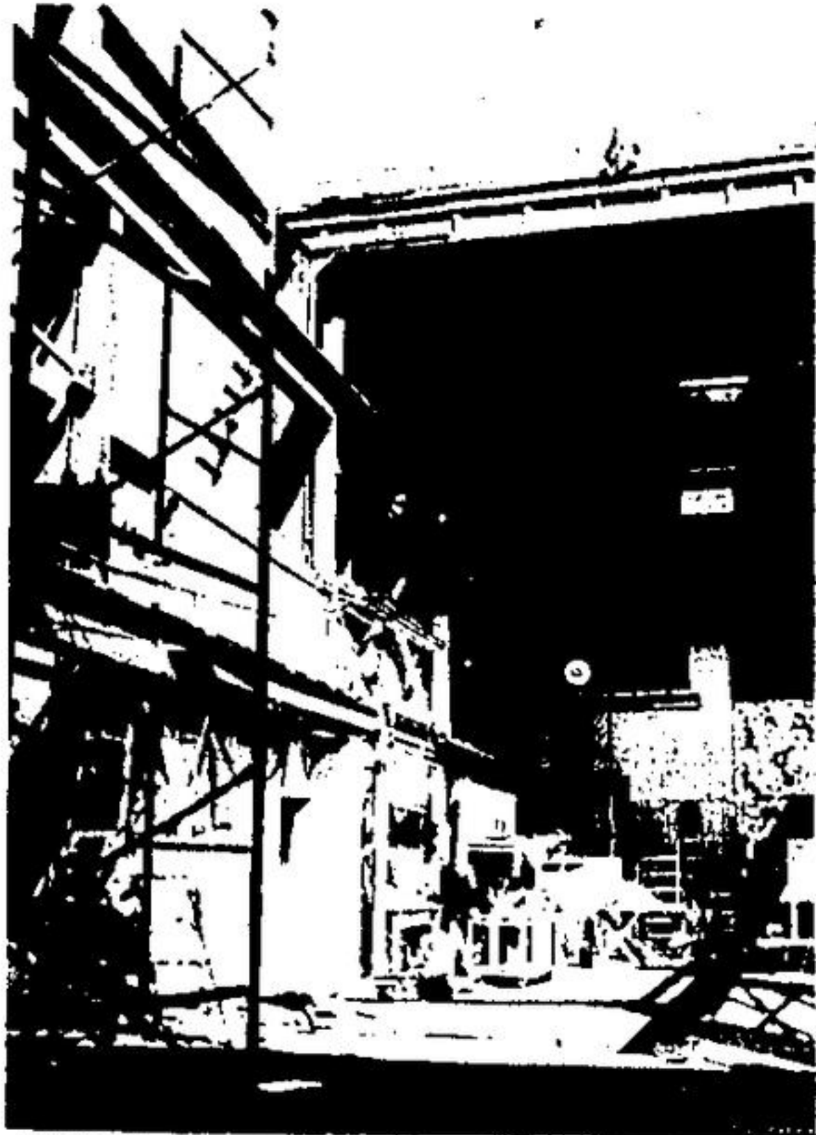
TWO NEW TALL bays are being added to Blow Press' operations. Work is expected to be completed this week.
