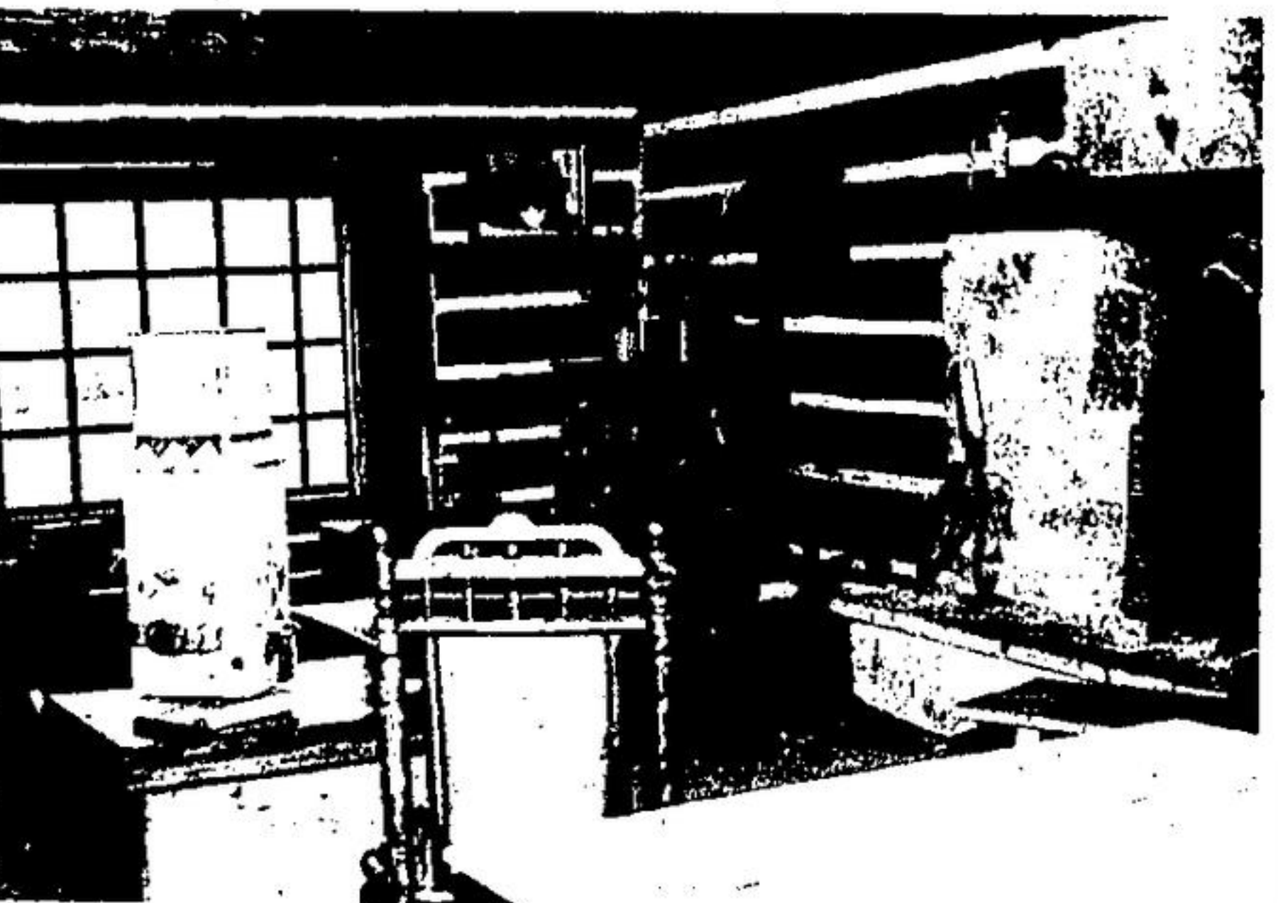
FILLED WITH ANTIQUES, the McMillan living room features white mortar between huge squared timber logs in the "piece en piece" construction of yesteryear.
