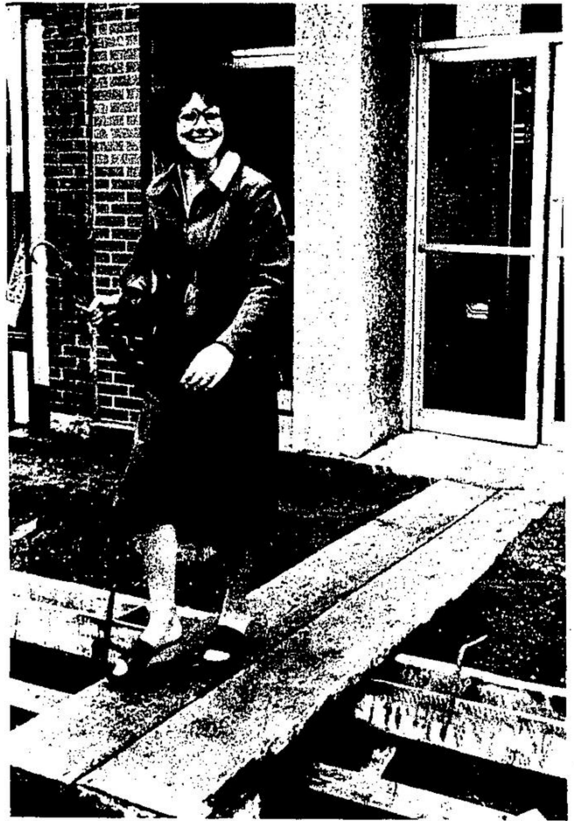
WALKING THE PLANK: Sue Buchanan picks her way along the boards which construction crews put up Thursday. Bridges allowed customers to get into shops while work goes on along Mill St.
