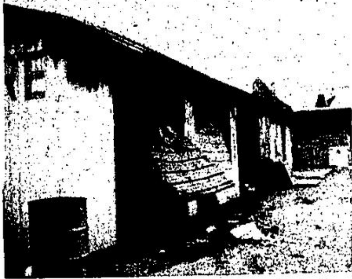
SECTION of building completely gutted when fire ravaged John Salmon's Country T.V. Centre early Tuesday morning, contained shipment of new appliances.
