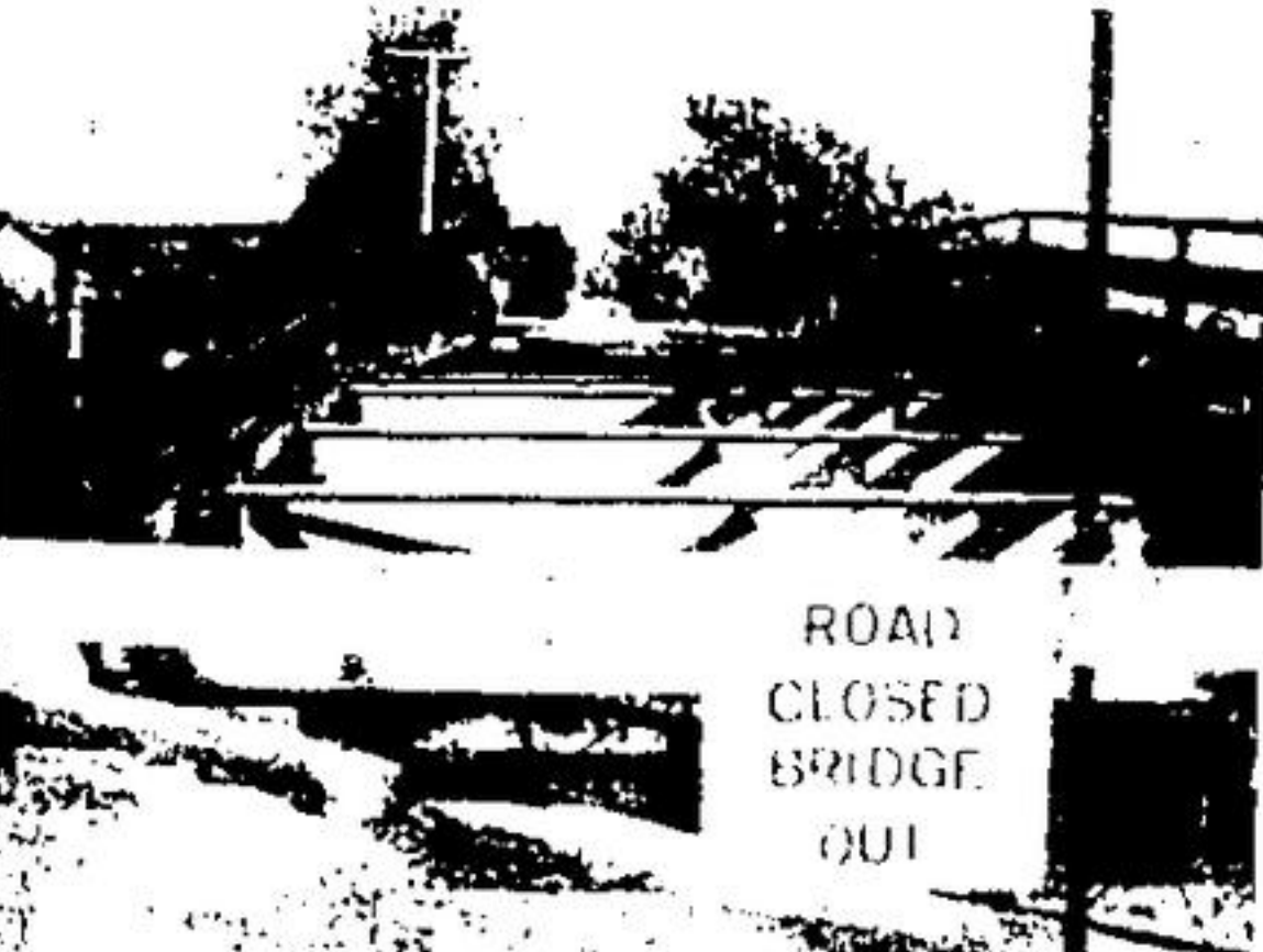
C.N.R. IS busy working on this bridge on the 6th line of Eramosa Township. This six-week job is nearly over and should be completed by the middle of June. The bridge is being replanked and strengthened for a heavier load limit. In the meantime area residents are somewhat frustrated.
