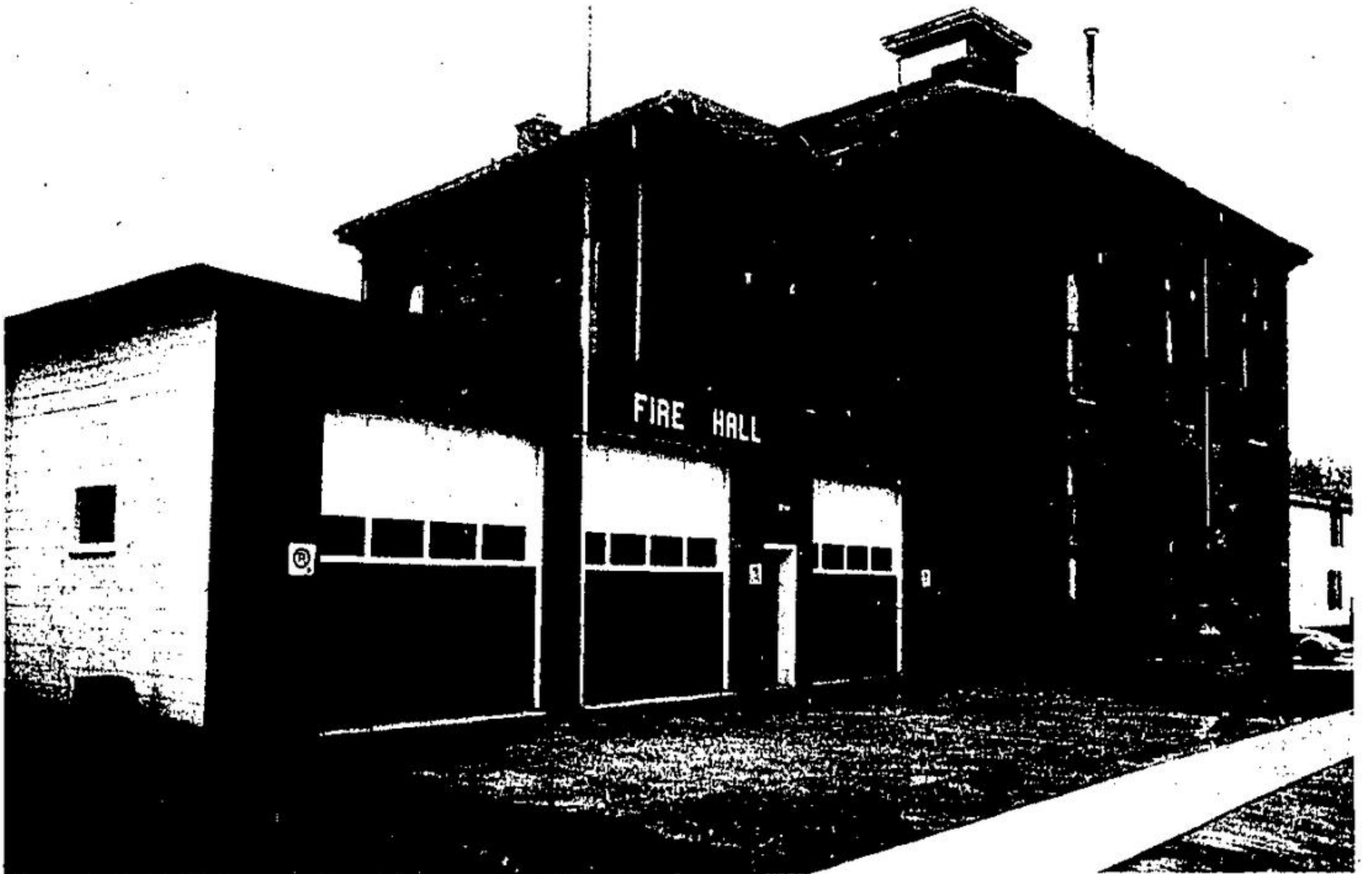
IF TOWN HALL were demolished, present fire hall could accommodate a full second storey. The stage area of the hall juts over the present hall. Council's works committee recommended last week the town hall be demolished to allow the extension and provide more parking. Feeling citizens were not given enough
