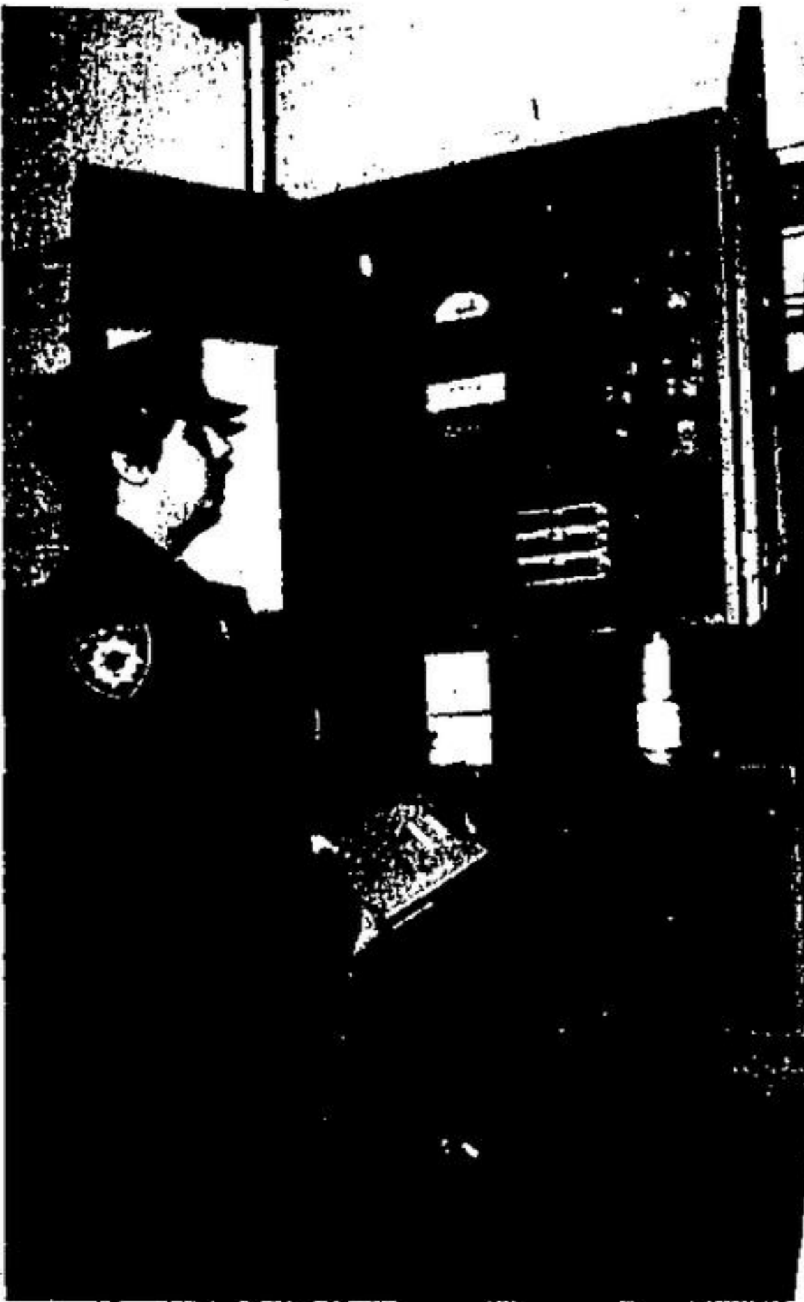
ELECTRICAL PANEL inspections are routine for Fire Prevention Officer Larry Bassard. He is presently inspecting all businesses and plants in Acton.
