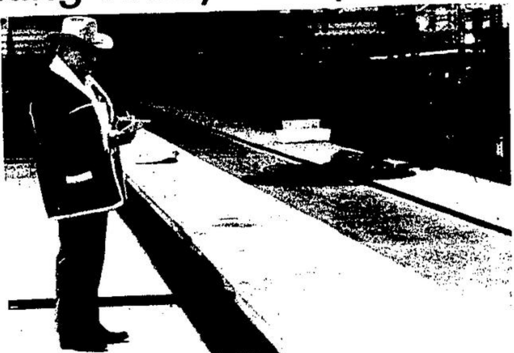
DON TOMLINSON checks the progress of the construction in Rockwood Gardens' new building. The building will help the company in its expansion, providing more working and storing space.
