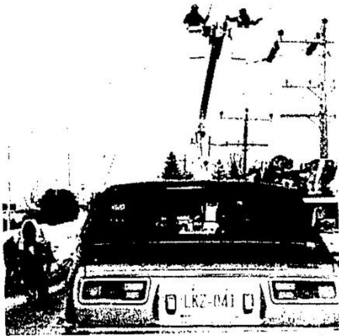
HYDRO WORKERS stop traffic as they install a new line on Highway 7 between Acton and Rockwood.
