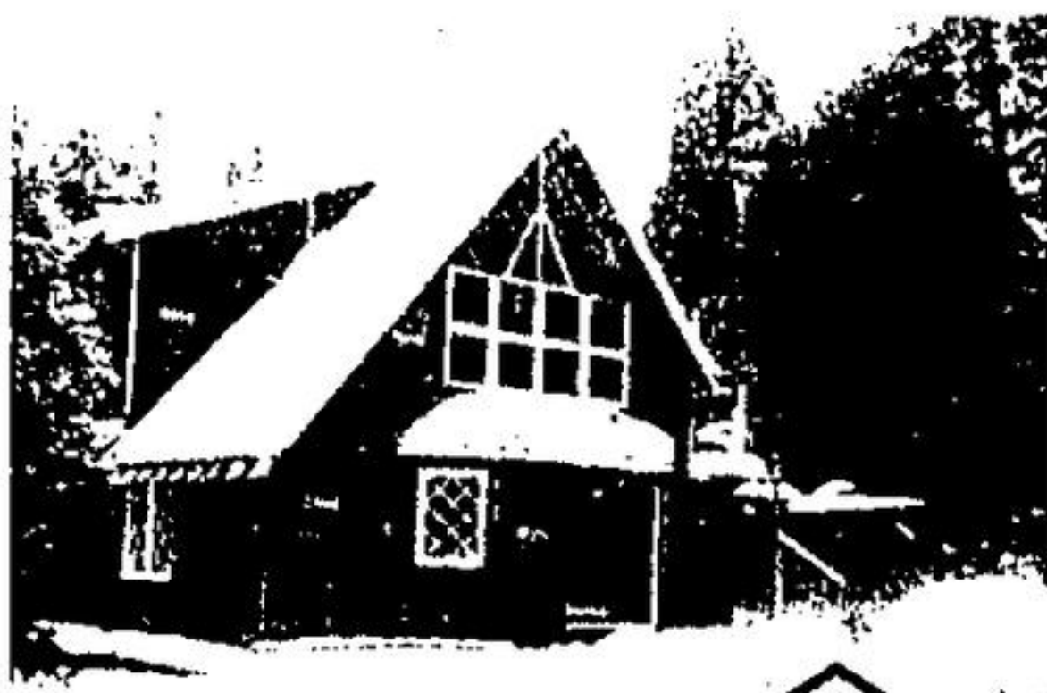
ARROW INDICATES what is left of original cottage. The McMullans intended to use the materials from this cottage for the exterior of their new recreational home.
