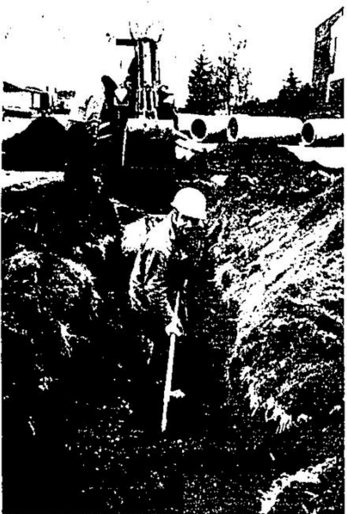
WM. HOSSINGWORTH AND SONS Ltd. started installation of 27-inch wide sewer pipe that will join Churchill Road to Acton Blvd. last Wednesday. The approximately $60,000 project stretches across the school yard and will take about a month to finish.
