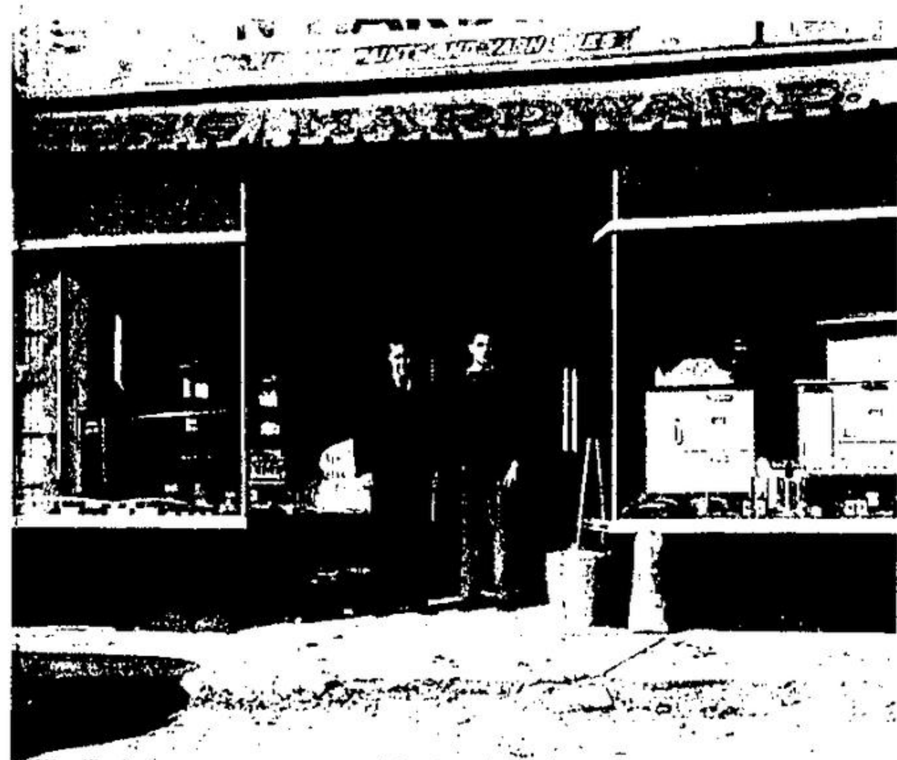
WHEN NEW SYMON Hardware store was built in 1935 Acton's first gas pump was taken off the street. However the pipe for filling the underground tanks remained, showing in the sidewalk on the right. Mac Symon and clerk Rod Ryder were pictured about 1942. A dentist had the upstairs office at this time. Rod Ryder was killed in an accident in 1949; Mac Symon sold the business to Mike Kinal.
