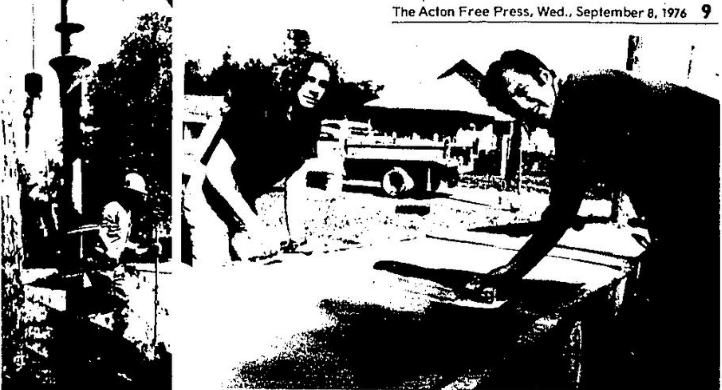
TOWN MEN ALLIN BOWEN (right) of Acton and Dave Majury of Georgetown smooth over freshly-poured cement on Mill Street West last Thursday. The new sidewalk is about three feet closer to the lake.
