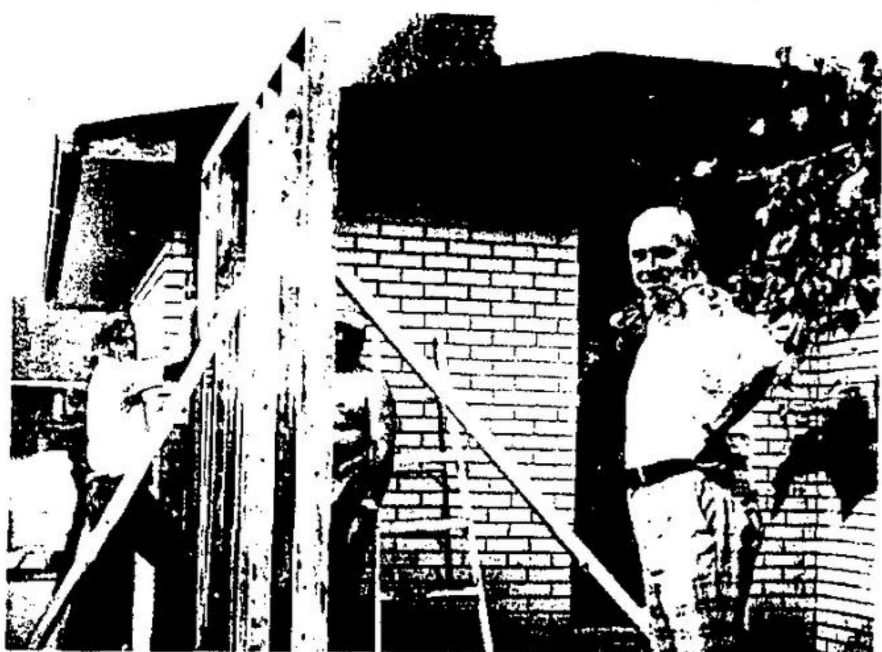
SUPERVISING THE NEW ADDITION to his house on Jeffrey Avenue, Dr. Oakes watches Vern Koreck and Ron Hiller at work. The addition will house a work shop for the Acton veterinarian now that he's officially retired, and has more time for the garden.
