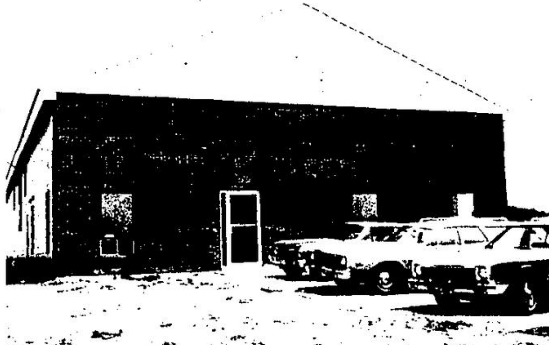
VACFORM'S BUILDING ON Commerce Court is the newest in the industrial complex north of the CNR Tracks. The company started production at the beginning of August after it moved from Mississauga.
