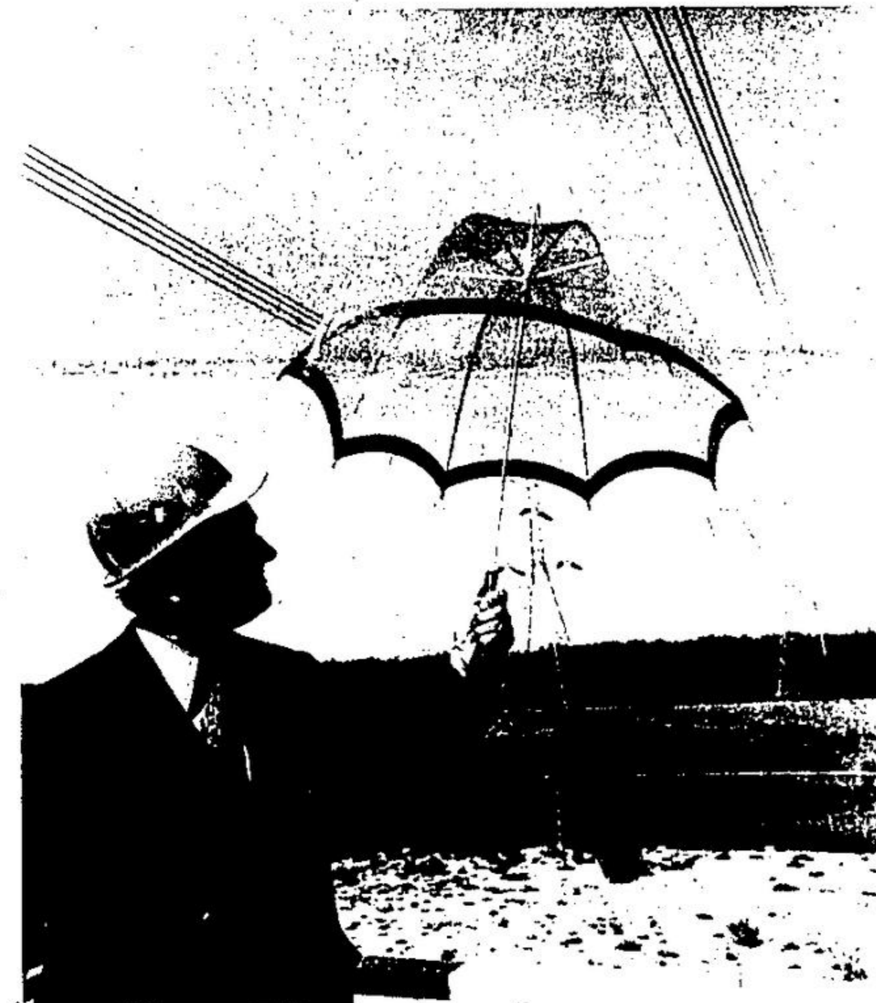
ELECTRIC FIELDS exist under 500 kV lines, Ontario Hydro admits, but claim they are low at ground level and cannot normally be felt. Walter Inkis demonstrates a slight tingle can be felt when an umbrella is used to magnify electrical effects.
