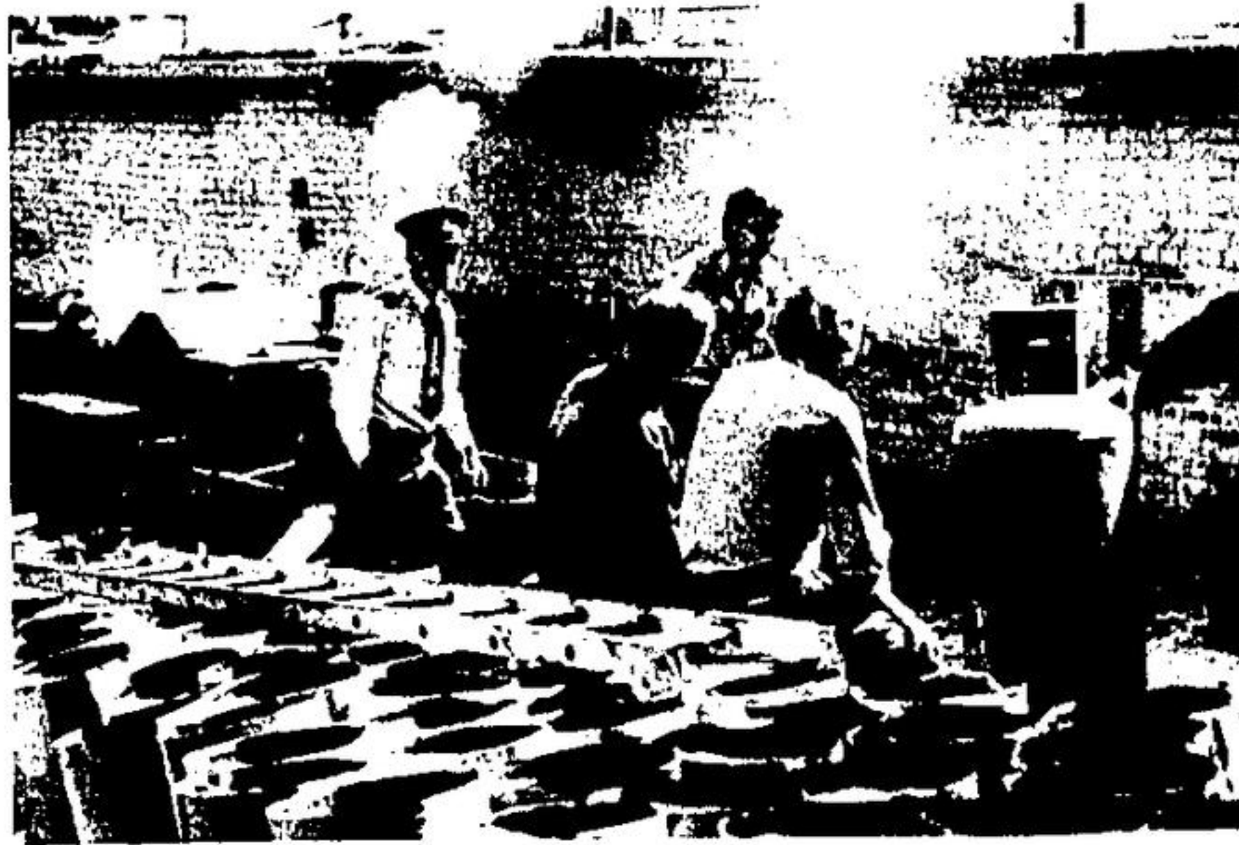
ACTON VOLUNTEER FIREFIGHTERS were called to Beardmore Thursday morning to extinguish a blaze in a tar pot. Contractors were tarring a roof when the sticky stuff ignited.
