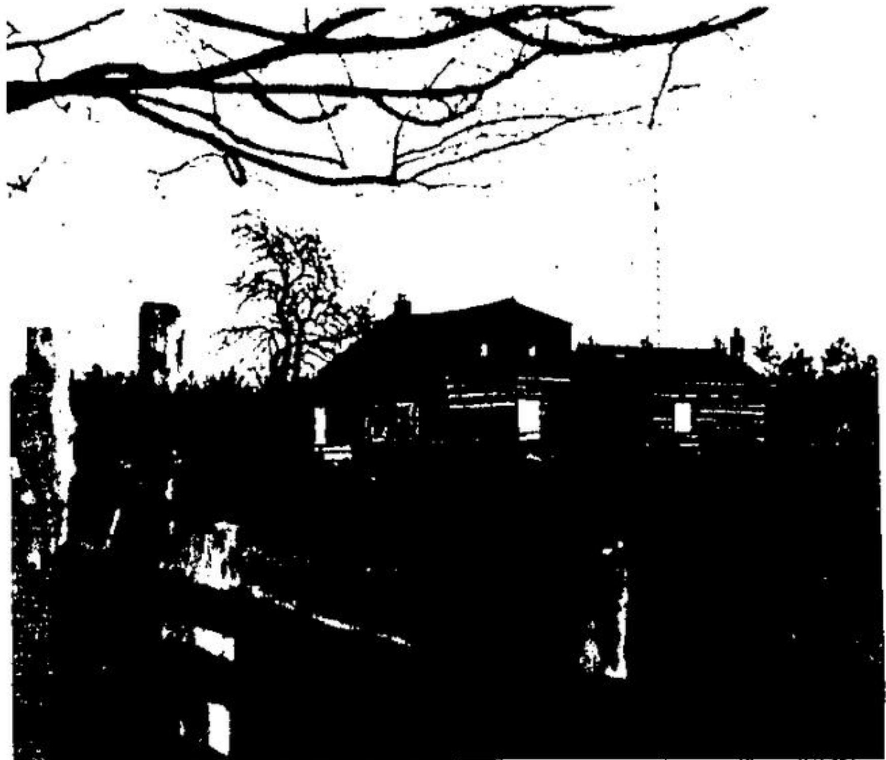
THE NEW TOPS OFF the old on a country road. A television aerial rises above the roof of a log cabin.
