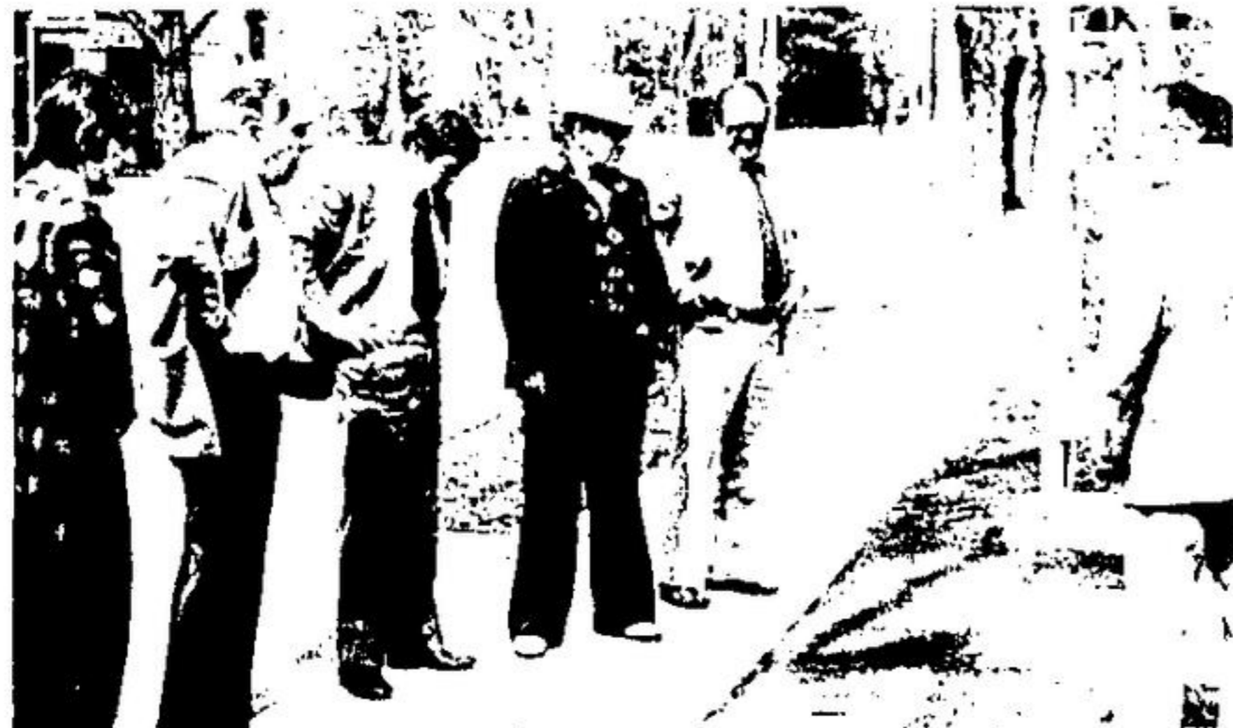
DEPUTY ENGINEER Ted Ballinger, Councillors Ern Hyde, Mike Armstrong, Pat McKenzie, Dick Howitt and Joe Hurst inspect a problem at the driveway of Charles Heard on Church Street, Acton, where water is settling because the sidewalk is too high.
