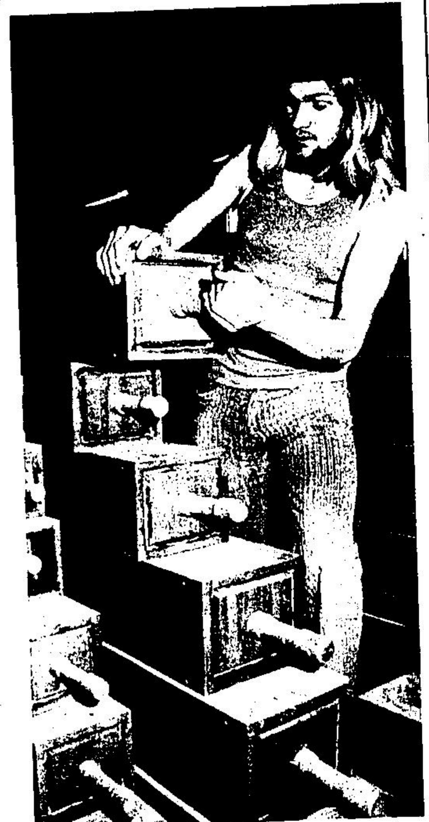
Ken Zeigler works on the hand-made 16 foot Bourdon pipes.
