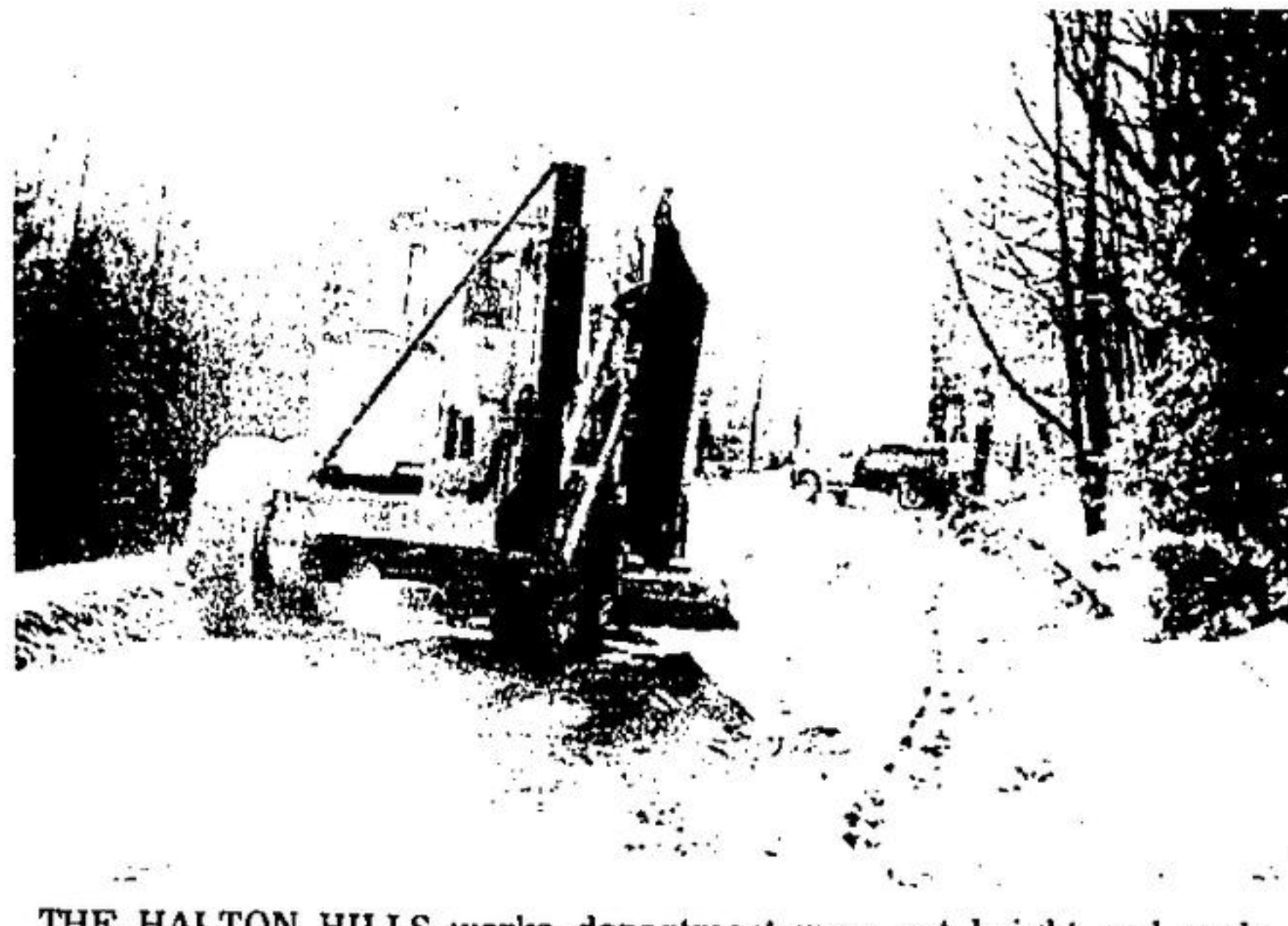
THE HALTON HILLS works department were out bright and early Thursday morning scraping down the fourth line road.
