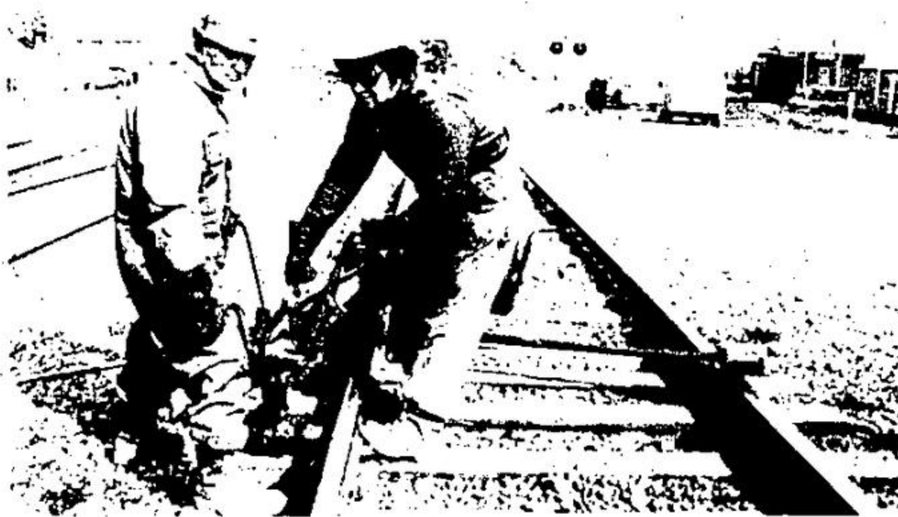
CNR maintenance crew members Louis Szabo, left, and Diego Vitello employ a bolt changing machine to replace insulation for the signals at the Mill Street West crossing in Acton. The project, performed by a crew numbering about 10, is part of annual maintenance.
