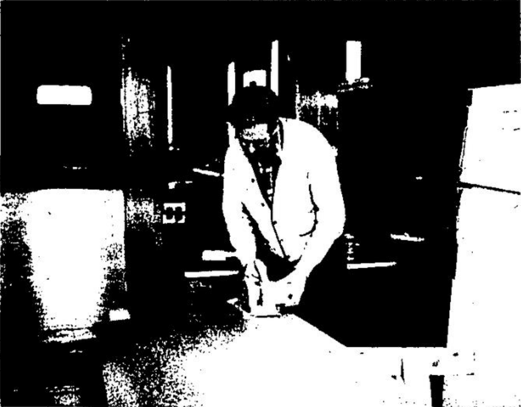
"STRAW BOSS" Murray McLaren prepares panelling for the new washrooms in the town hall. He is assisted by Murray Haig (not available for photo) who did the excellent job of drafting for the project. The two men have undertaken the town hall renovation and beautification. Trustee Pat Smith is responsible for the overall administration of this undertaking.
