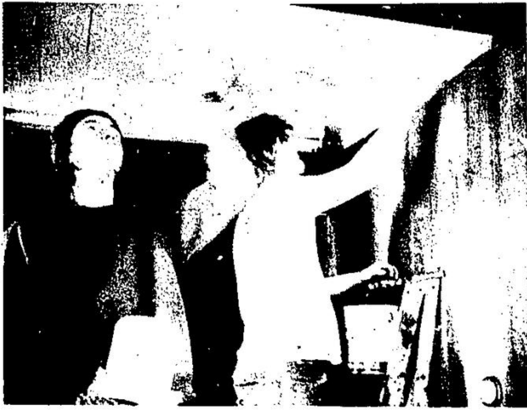
BUTCH GIVEN and Peter Bolton, the demon painters, apply the finishing touches to the new ceiling outside the men's washroom in the town hall. The boys were employed on a part-time basis to assist on this LIP project. Much of the work done up to this point has been underground, the building of a furnace room and the fire-proofing of the back portion of the building. Village residents will soon see some changes as the renovation moves ahead on the main hall and exterior.
