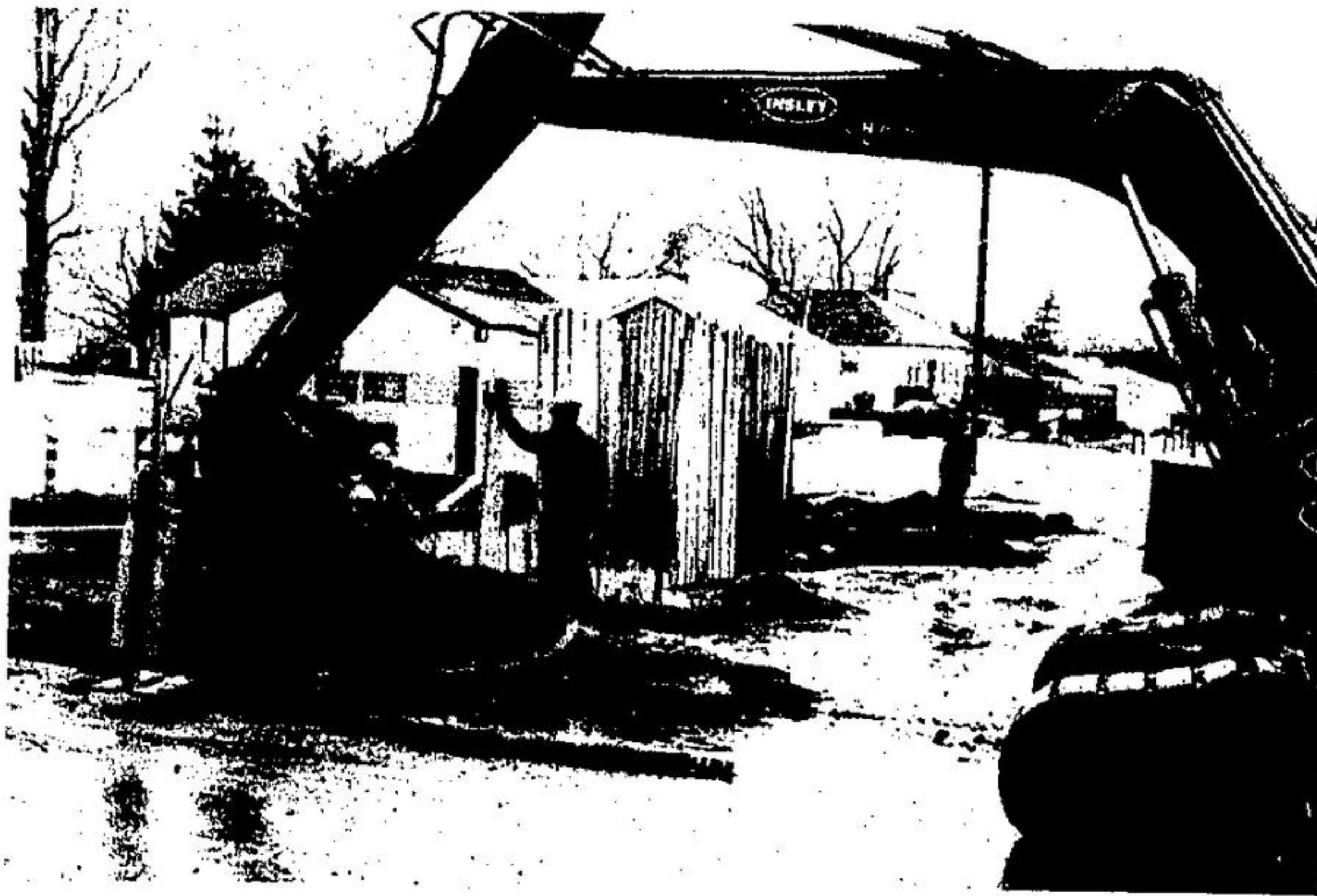
SEWER WORK UNDER CAMERON STREET got underway Friday. Workmen have dug a long ditch reaching down between nine and 16 feet in sandy soil. The placing of boards side-by-side
