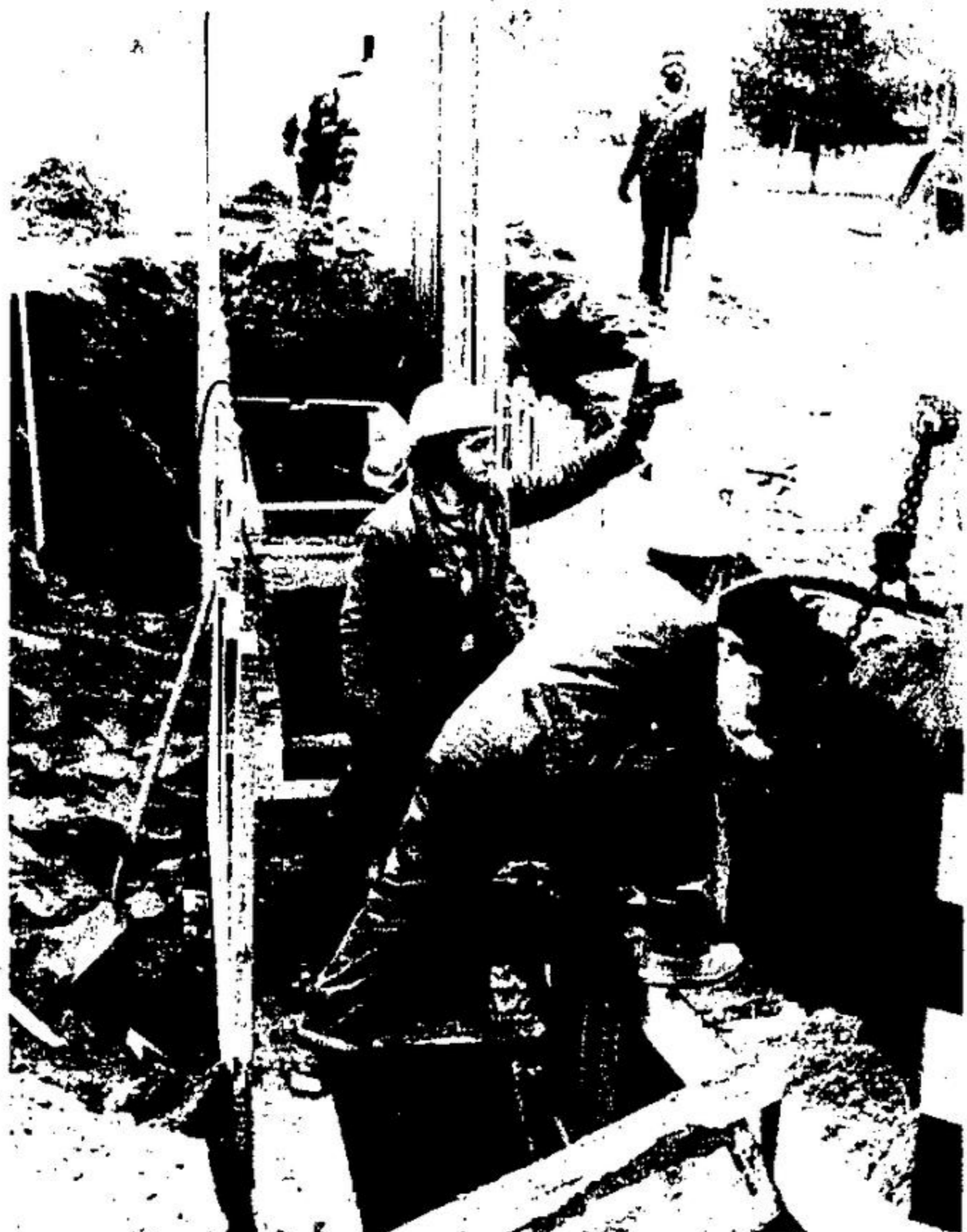
A WORKMAN SIGNALS to a powershovel operator, just off camera, to hoist one of the wood planks used to shore up a sewer trench in Cameron Street. The digging is heading north toward the lake, and is expected to take three weeks before the work is completed. Hidden from the camera's view are the workmen toiling several feet below the surface.
