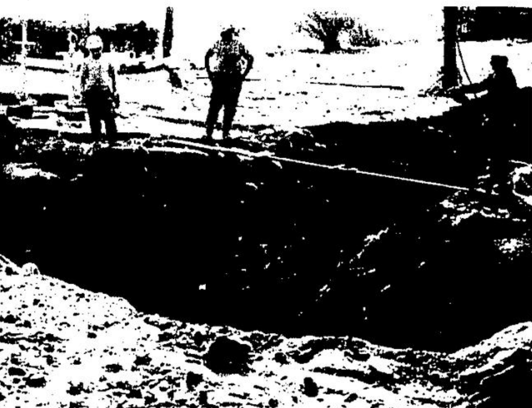
THE SUPERVISOR ON THE RIGHT could be telling workers on the Rockwood sewer and water pipe project to keep a wary eye open for signs of other tunnellers working their way north from Metro. Subway workers are digging under Spadina Avenue in Toronto to add a few more miles of underground track to the transportation system, while the Rockwood installation will be heading to the southern part of the village. A linking of the two projects, while possible, is highly unlikely.
