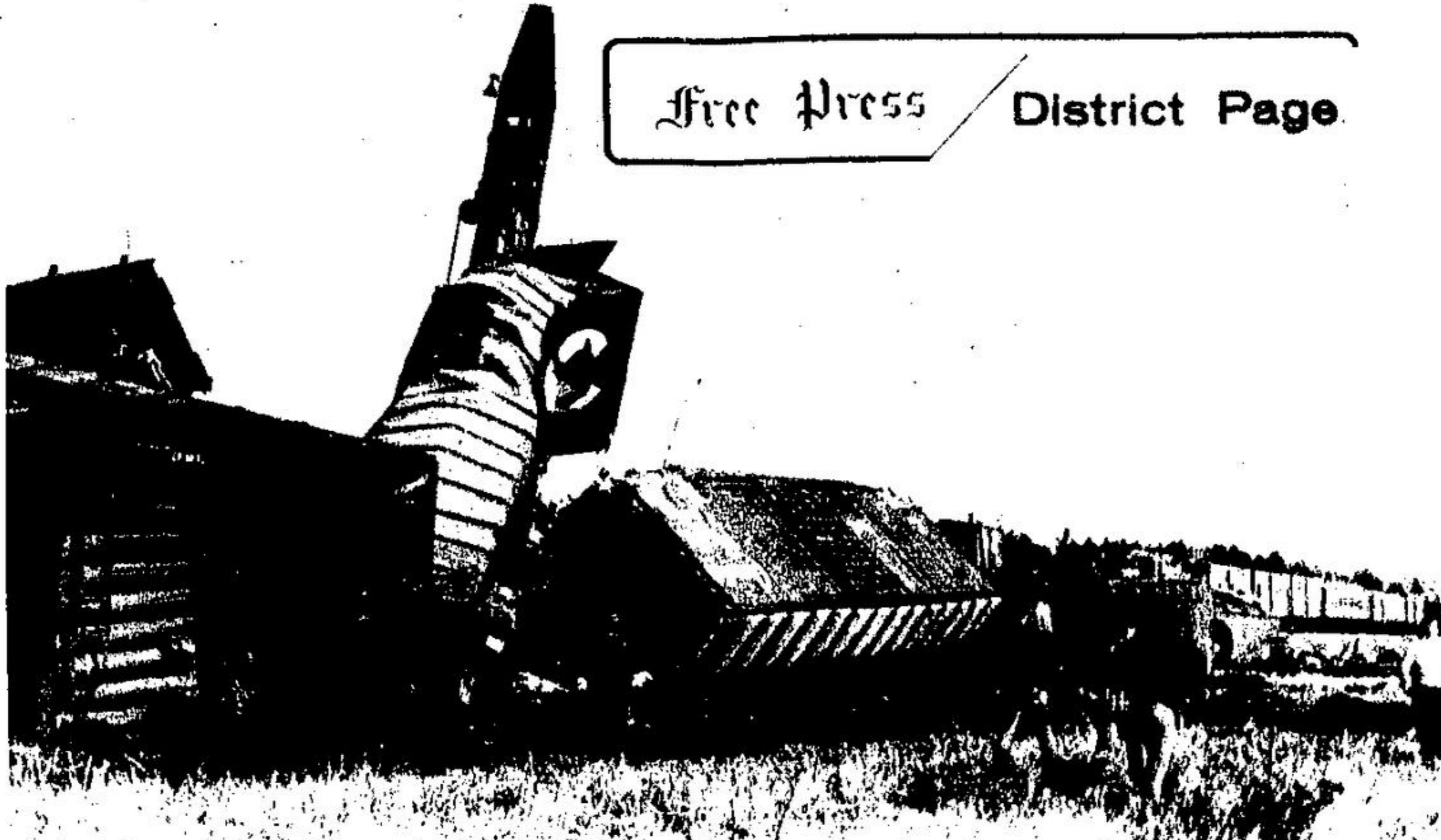
GIANT CRANES were used last week by CP Rail recovery crews to untangle the 40-odd freight cars and two locomotives which plunged off the main line near Puslinch after the train hit a gravel truck at a level crossing. Two men died in the fiery collision and the major rail link, 20 miles west of Milton, was closed for the week.
