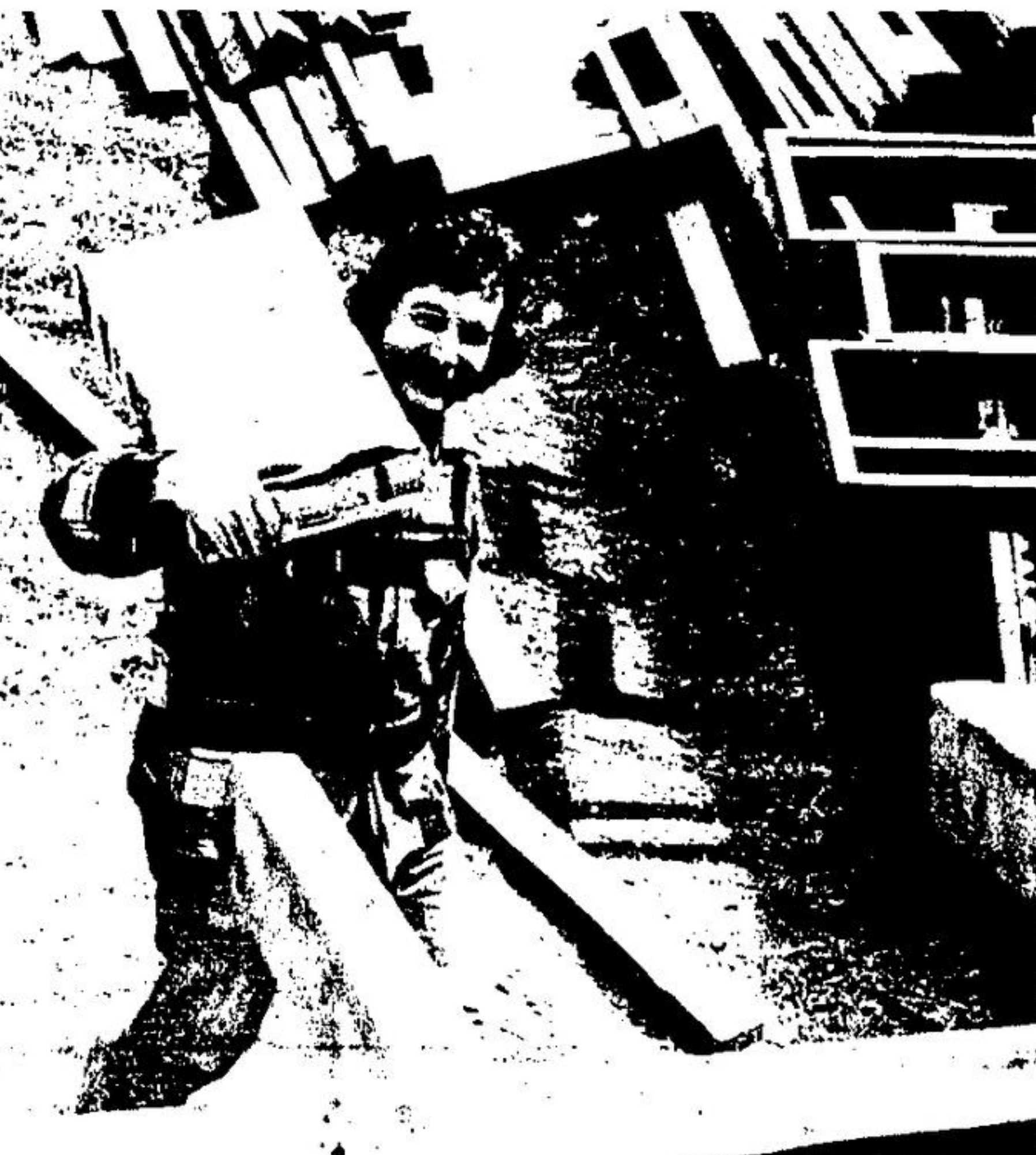
HANDSOME volunteer at the scout hall addition site Saturday was Bill Cook. He's good at selling ads, too. There have been work bees on the building every weekend lately.
