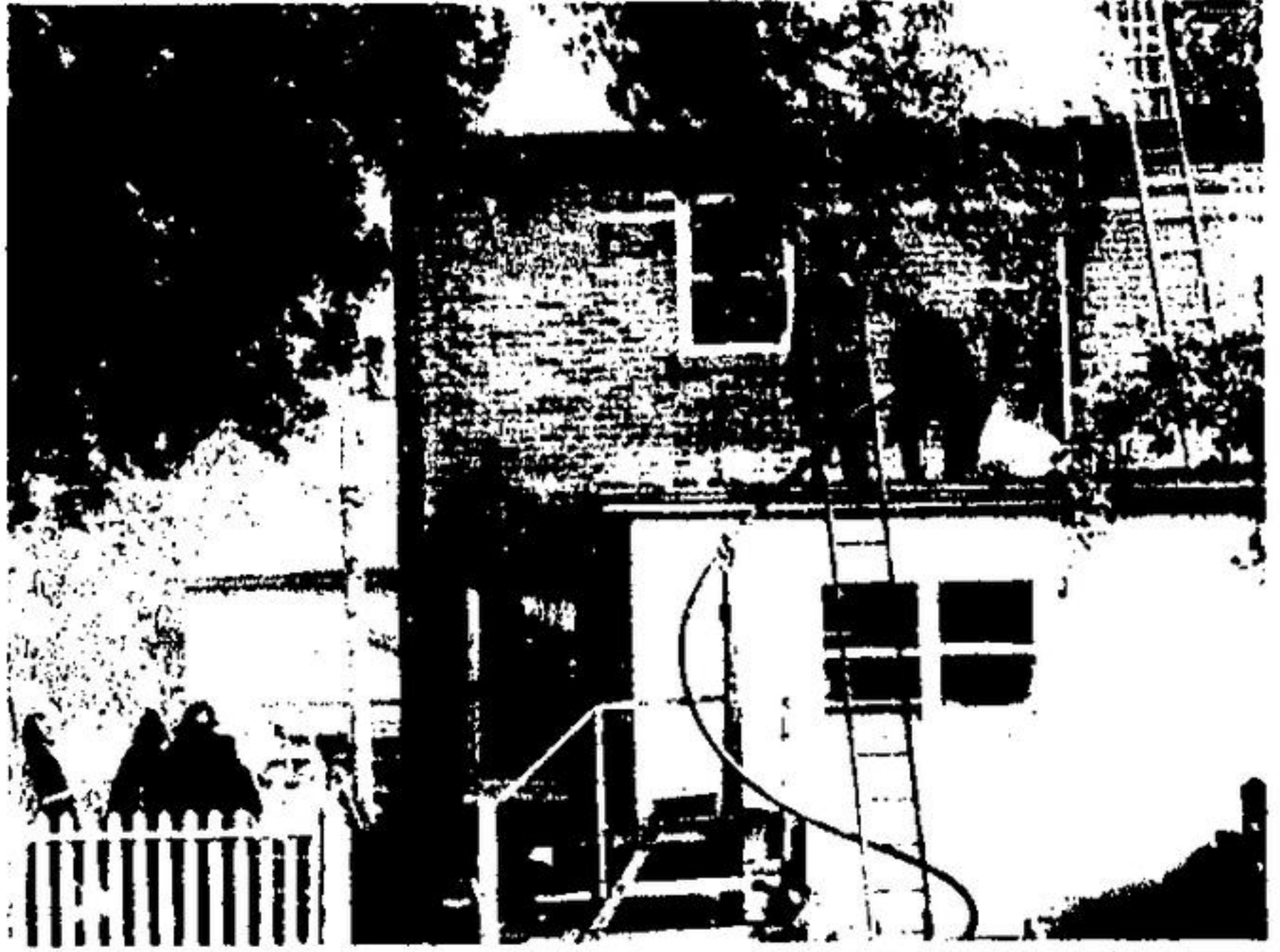
FIRE AT Bower Ave. home of Mr. and Mrs. Paul Braida started in upstairs bedroom. Burned material was thrown out of upstairs window by firefighters last Wednesday.
