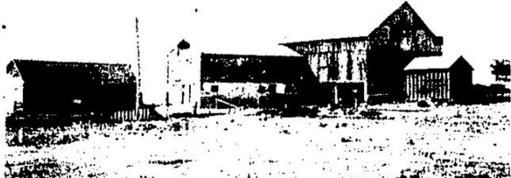
THE BARN AND DRIVING SHED on the farm known for many years as Edgar Beene's was razed recently to make way for Joe Prucyk's home and is now the site of a snack bar at Waterfalls Park.
