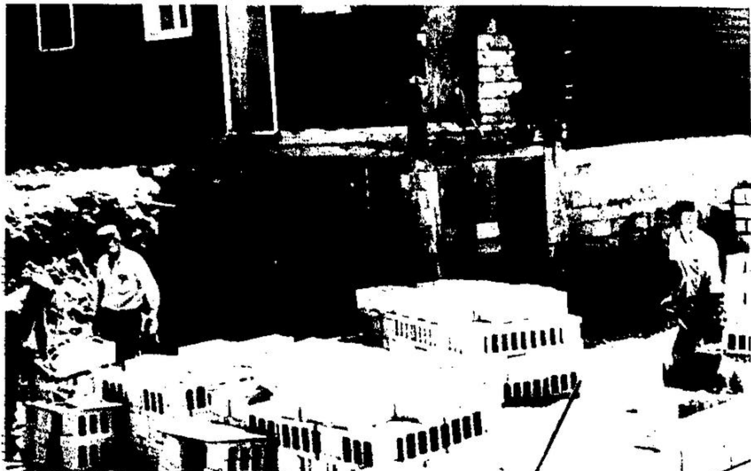
PROFESSIONAL masonry contractors who donated time last Saturday and Sunday have been loudly applauded by Rotarians sponsoring the scouting movement. Murray Hurgett, Les Trevail and Fred Allen were the local experts who worked on the basement addition to the
