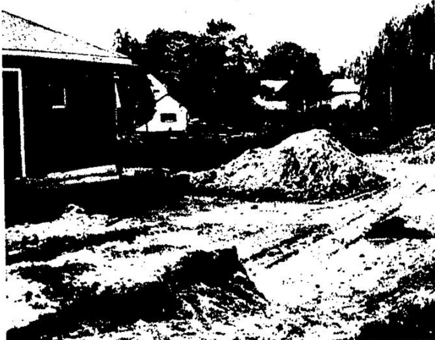
ACTON SCOUTS and guides will have expanded facilities by September. That's when construction of the new addition is estimated for completion. The cost is between $5,000 and $6,000. The present building is being used seven days a week.
