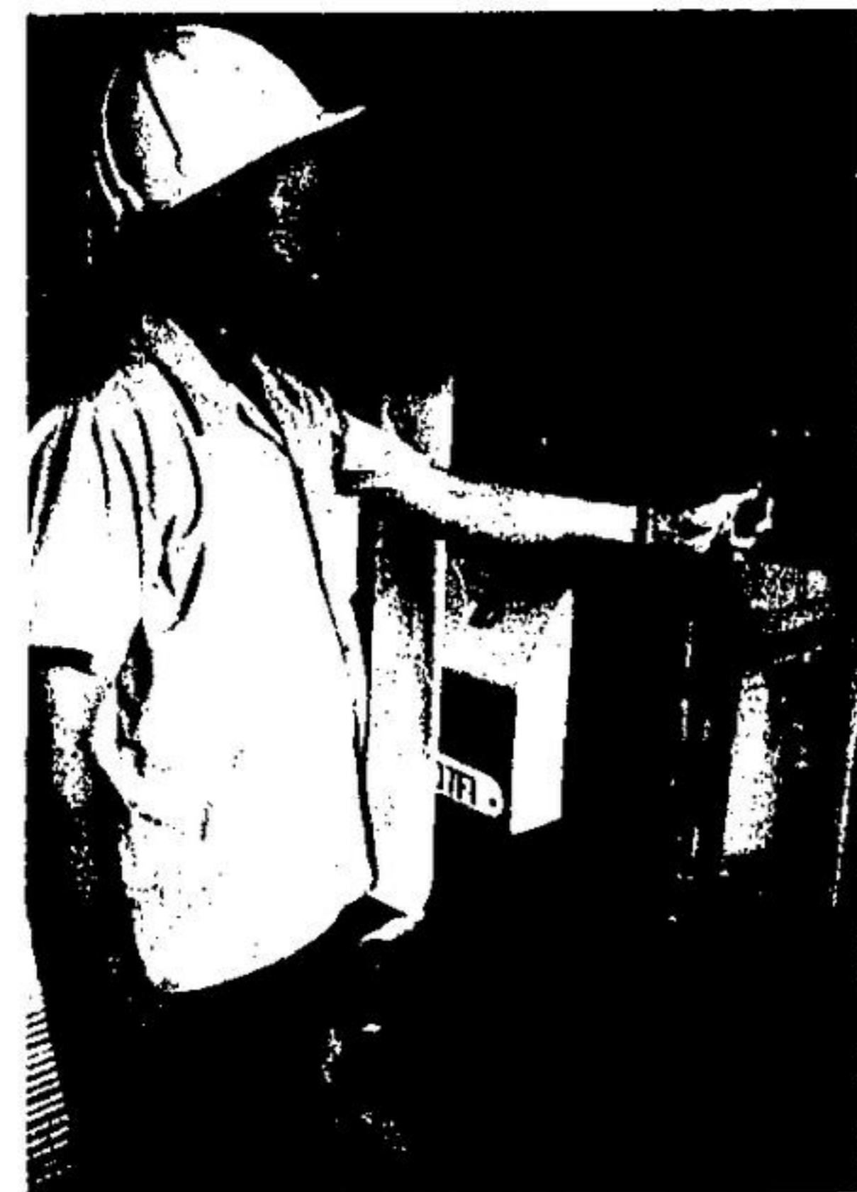
DOUG MASON switches the power on for the Church Street and Bovis subdivision areas of town which were without power part of Saturday and Sunday. A cup of hot coffee couldn't be had for several hours. The shut off was due to the Church St. reconstruction.
