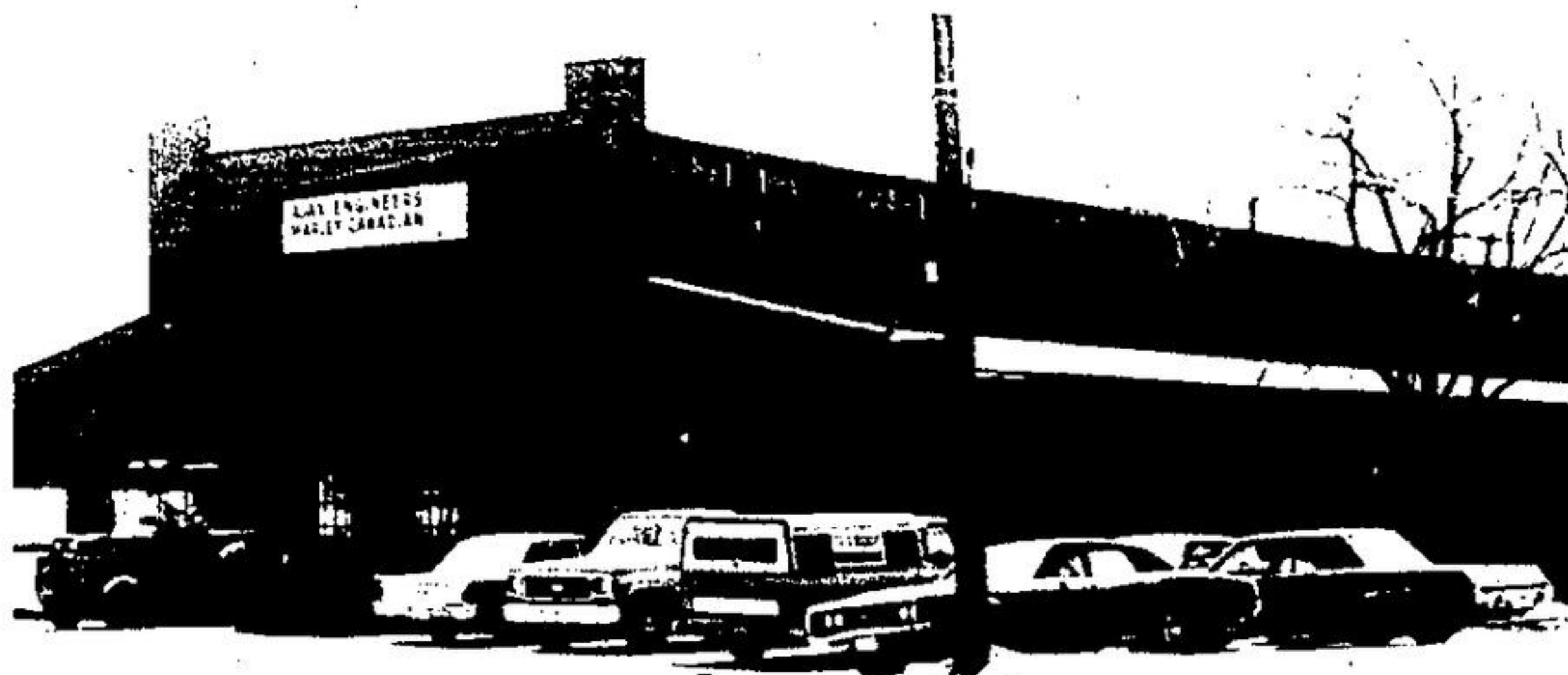
AJAX ENGINEERING plant was established in town on Queen St. in 1935. Radio towers were manufactured at first as well as cooling towers
