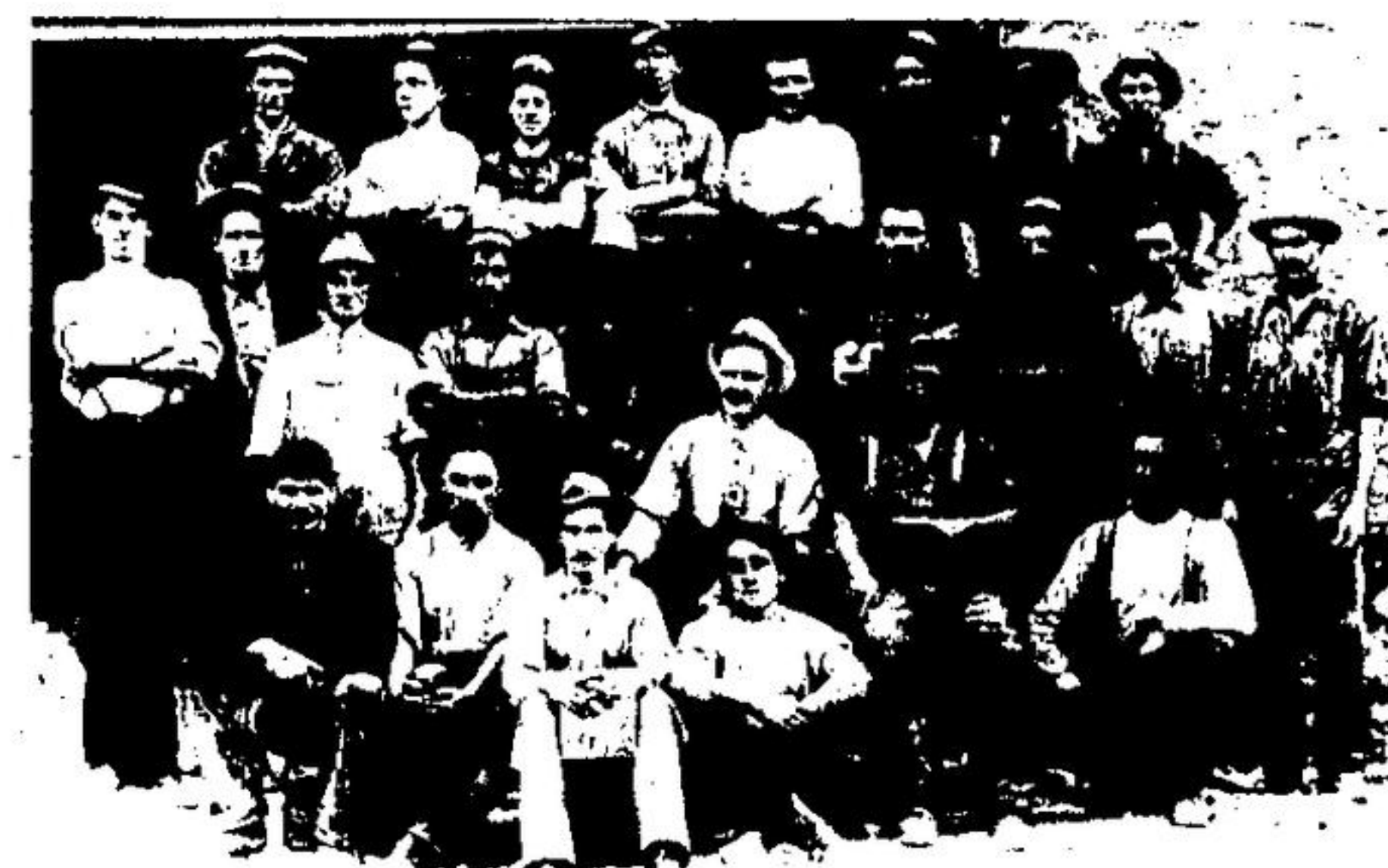
WORKERS AT the Toronto Lime Company at Dolly Varden near Limehouse in 1913. William Gowdy can be identified. He is sitting in the centre of the picture with white shirt and tie.
