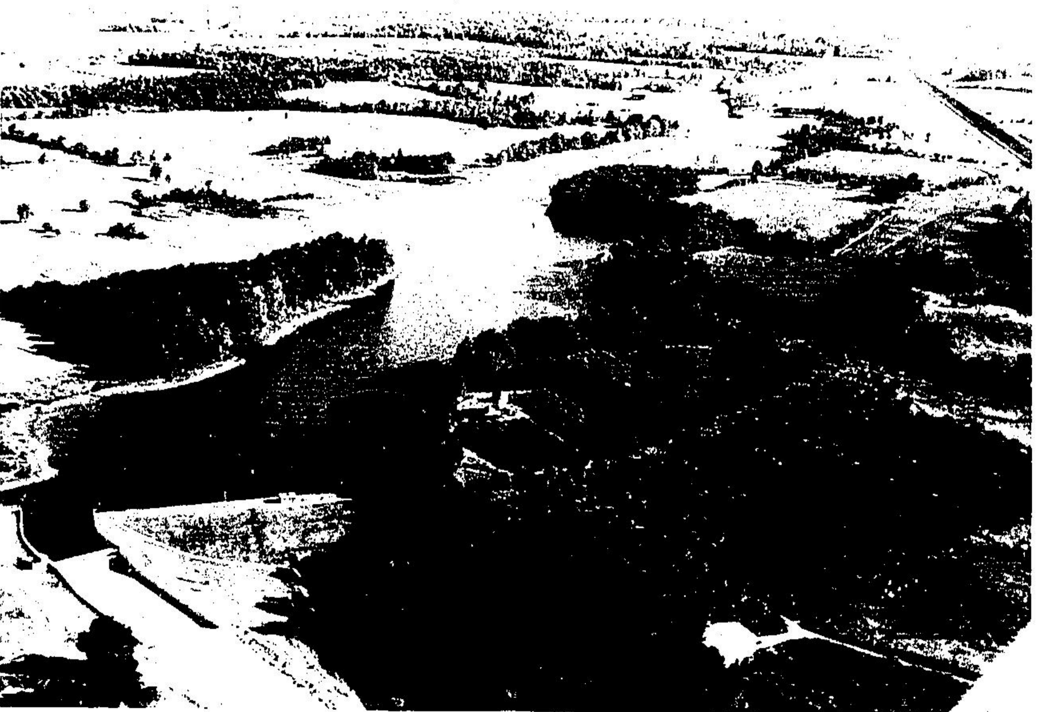
A VIEW from the air shows Scotch Block Dam in a scenic setting.
