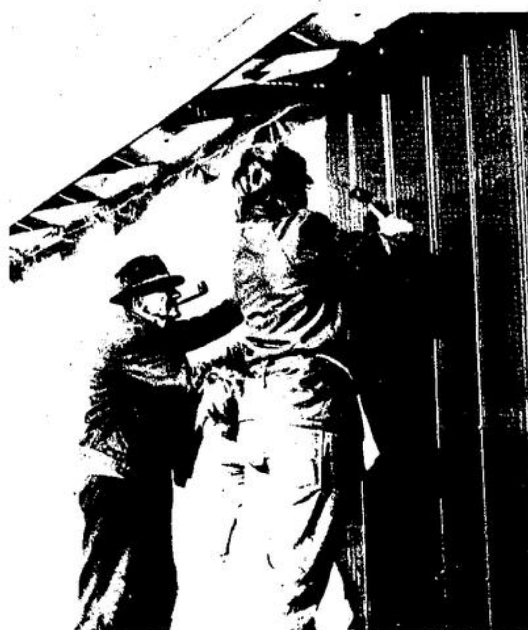
OLD-TIME CRAFTSMEN and young men eager to learn the trade are restoring old barns and building new. Here they put the aluminum siding on a new horse barn.
